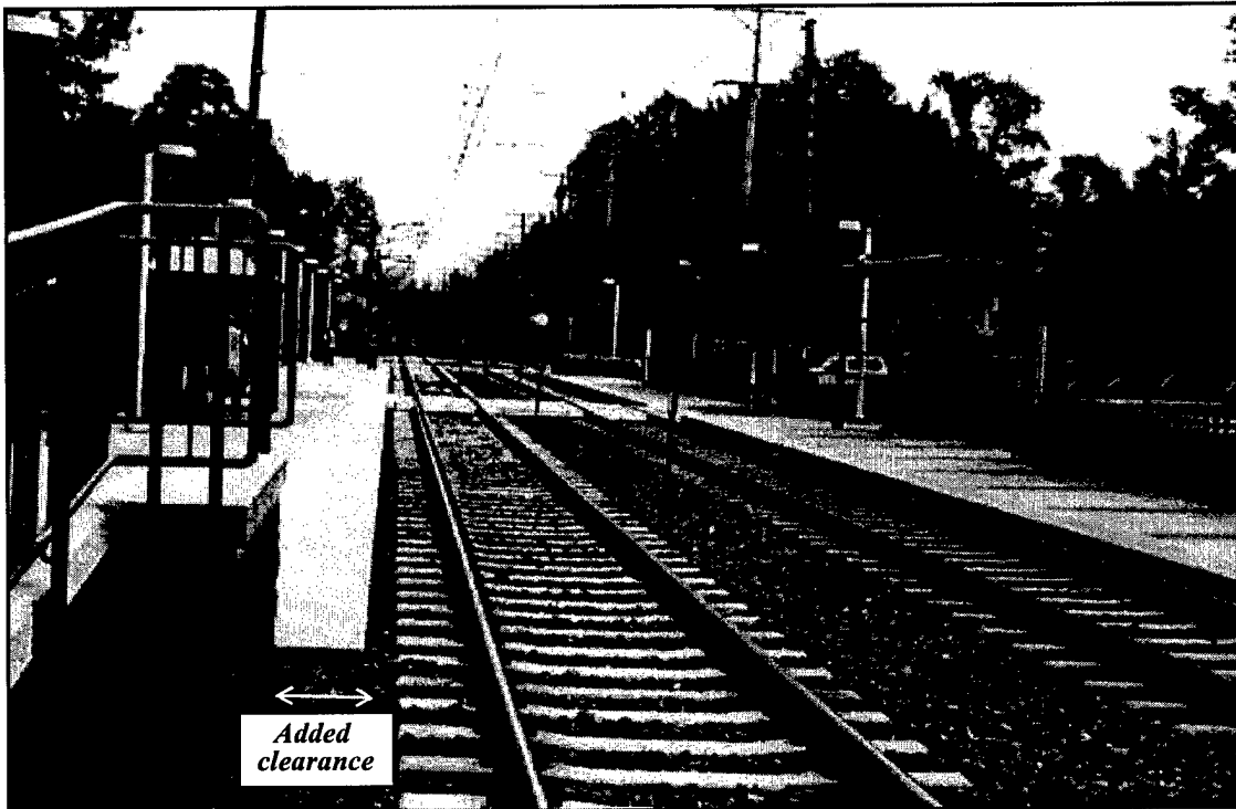
Figure 7. Offset Wheelchair Access Platform
