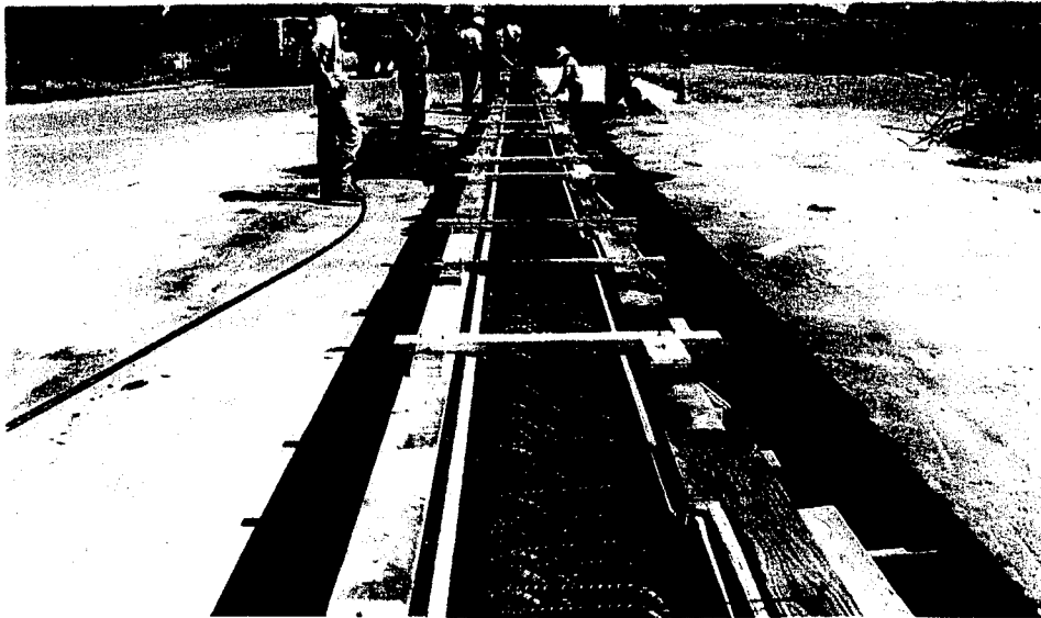
Figure 2-8 Top View of Forms for Beam Section
