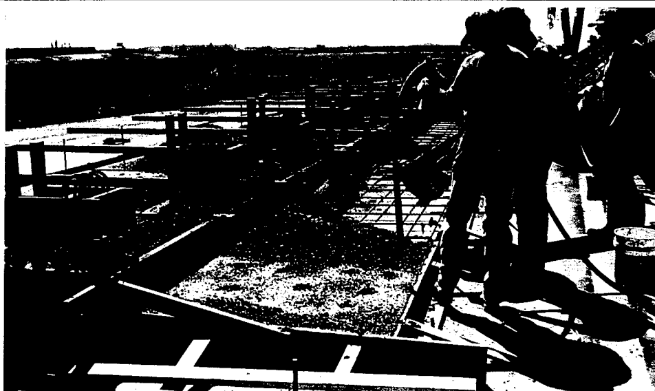
Figure 2-5 - Concrete Pour for Sidewalk and Curb Section of Bridge Rail
