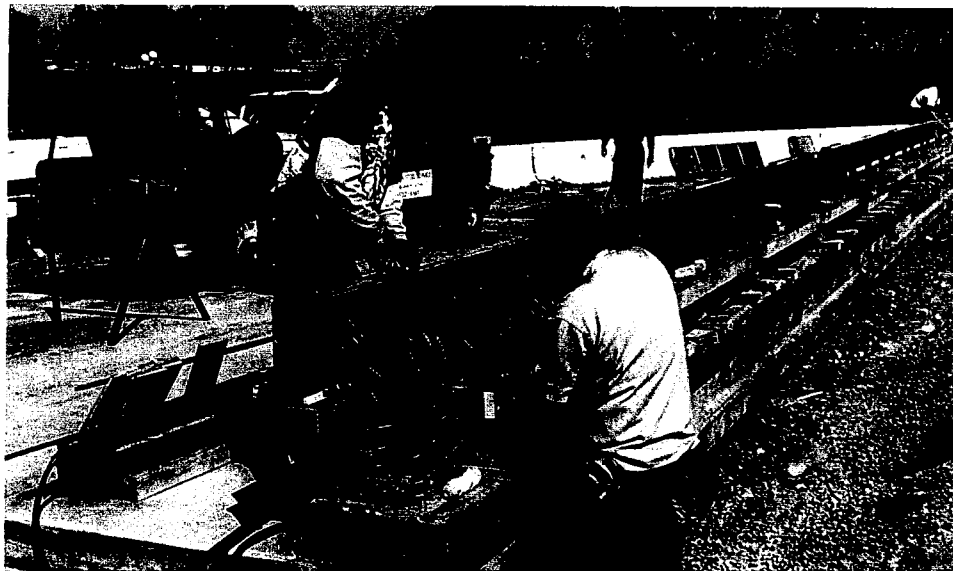
Figure 2-9 - Reinforcing Steel Placement for the Post and Beam Sections
