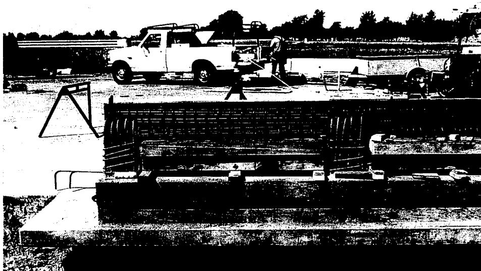
Figure 2-6 - Reinforcing Steel for Posts and Beam Section of Bridge Rail
