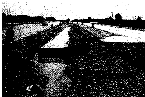
Figure 3: Sediment-control fence
