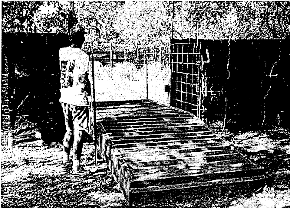
Fig. 8a. Sloped guard installed in cross fence at Welder Wildlife Foundation Refuge, Sinton, Texas.
