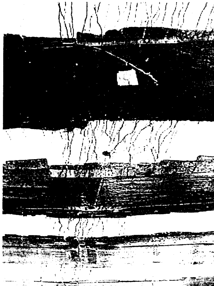
(a) Cracks on deck soffit
