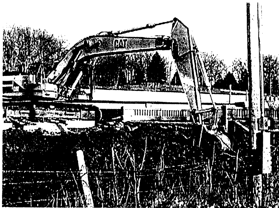
Figure 4.10. Excavating behind the bridge abutment.
