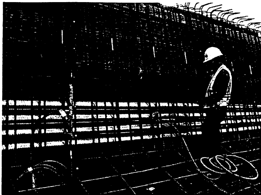
Figure 3.38: Embedment of a Strain Gauge During Construction at West Street On-Ramp
