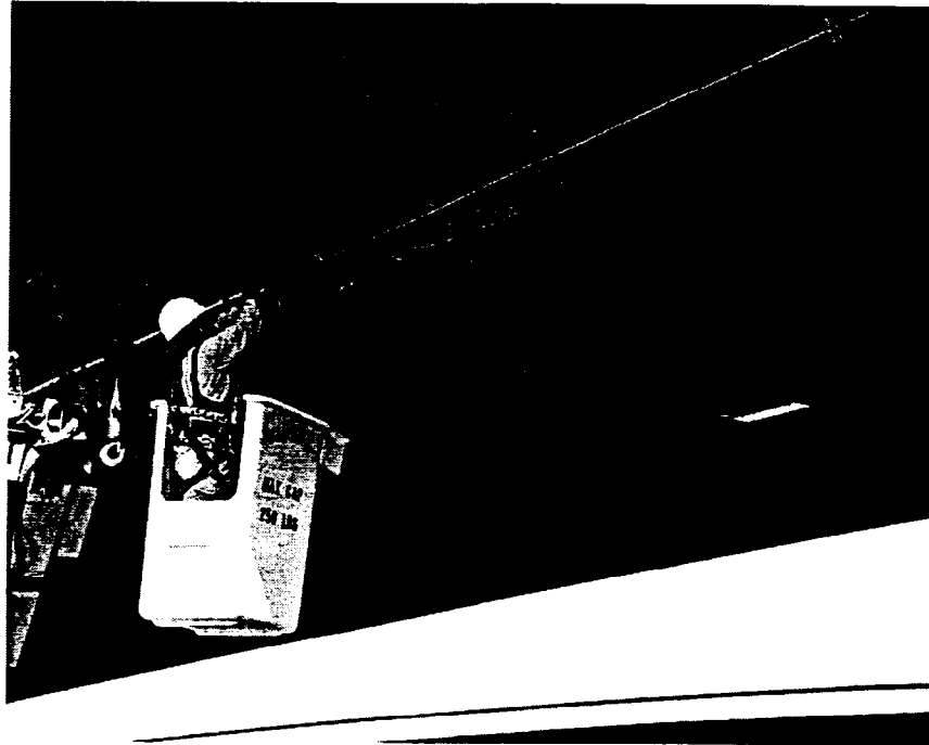
Figure 3.37: Installation of Cable Ducts Using a Cherry Picker
