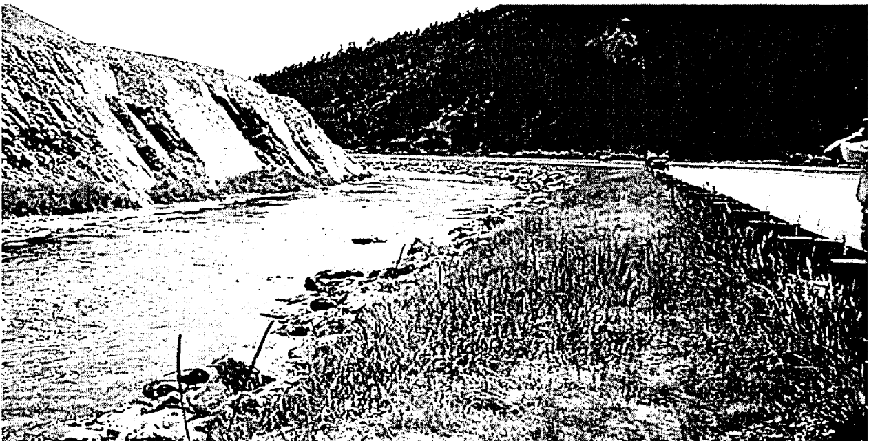
Figure 5. Interstate 90 and relocated channel of the Clark Fork River near Drummond, Montana. Note the lack of riparian vegetation and channel roughness elements. The river is no longer connected to its floodplain. High cutslope to the left of the channel reflects sunlight into the channel.
