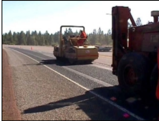
Figure 4.37: Compaction with Steel-Wheeled Roller
