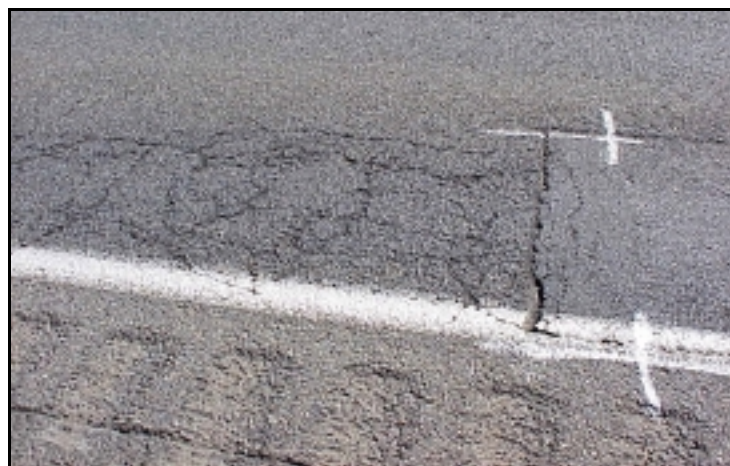
Figure 4.30: Distress at North Edge of Figure 4.28 Plug Patch, which Occurred after Patch was Installed
