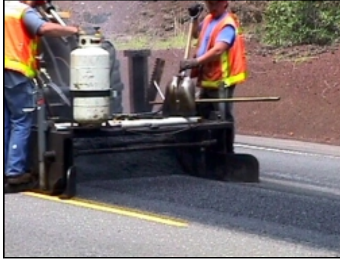
Figure 4.22: Close-up View of Screed Box and Windrow
