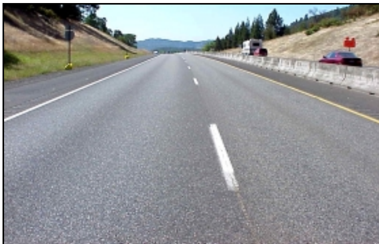
Figure 4.32: Full-width, 1.6 Km (approx.) Inlay of Outside Lane with F-mix, I-5 NB in Roseburg
