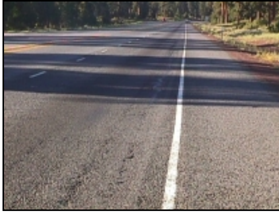
Figure 4.39: F-mix Distress at MP 148.4 SB prior to July 1999 Repair
