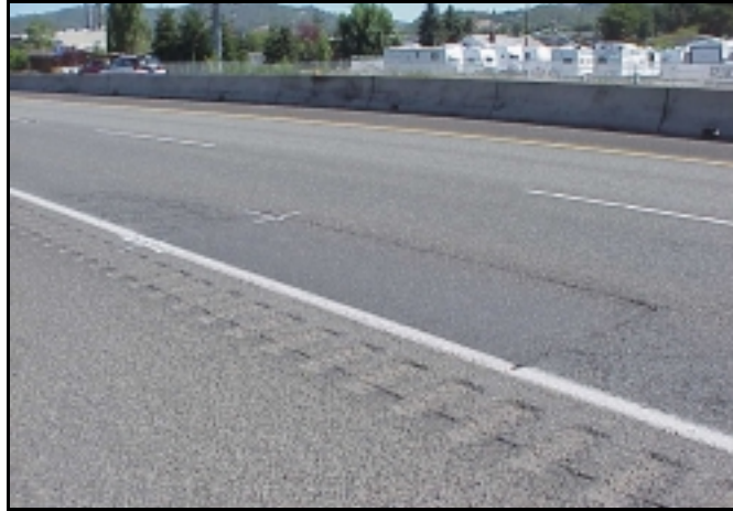
Figure 4.28: Plug Patch on I-5 SB in Roseburg
