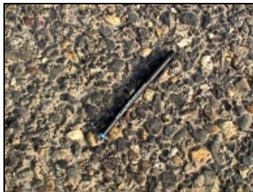
Figure 4.13: I-84, MP28 WB, Aggregate Retention on Shoulder, August 1999
