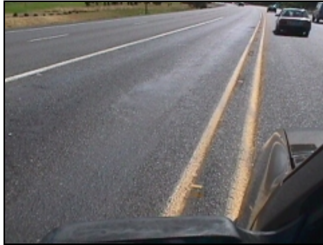
Figure 3.5: Deformation Rutting in WB Left Turn Lane from ORE 34 to Corvallis Bypass, August 5, 1999
