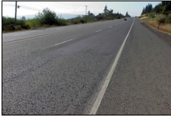
Figure 3.3: Raveled F-mix and Dense-Graded Blade-Patch on ORE 42, MP 18 (approx.) near Coquille
