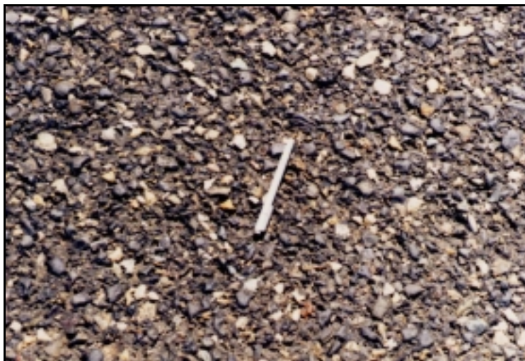
Figure 4.10: I-84, MP28 WB, Aggregate Loss in Outside Wheelpath, August 1997
