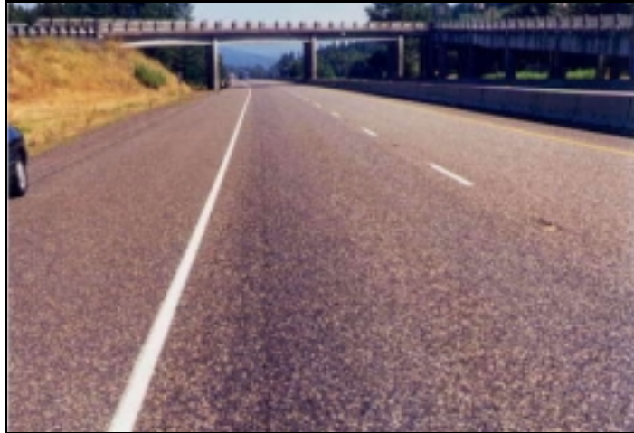
Figure 4.8: I-84, MP28 WB, Looking East, August 1997
