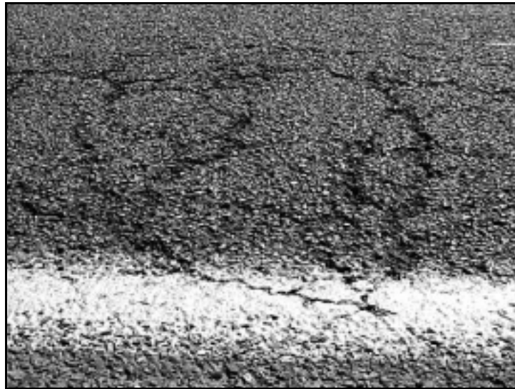
Figure 4.29: Distressed Pavement near Figure 4.28, Planned for Plug Patch Summer of 2001
