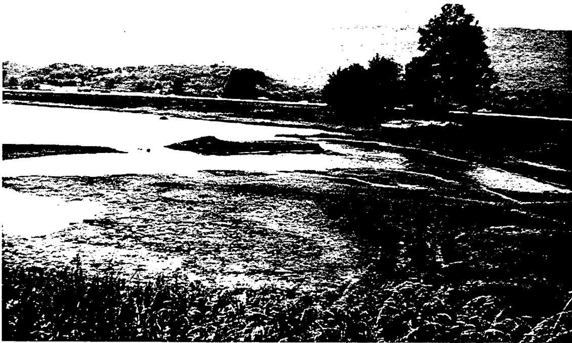
North end of Large Borrow Pit - August 1980
