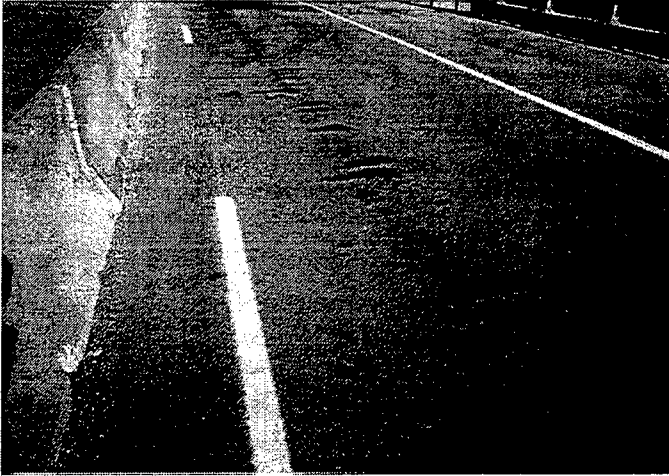
Photo 5: Pre-installation, westbound West Garrison.
