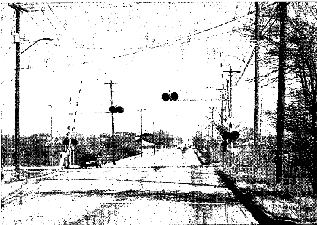
Figure 5-1. Picture of a Typical Crossing.
