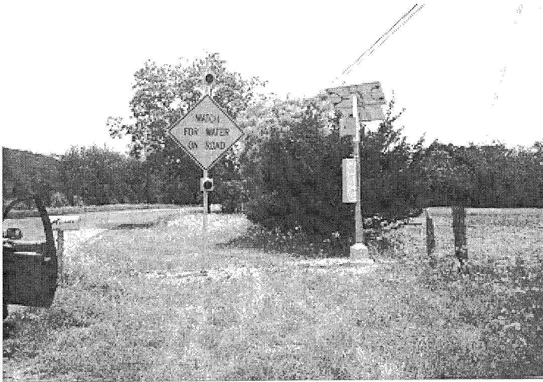
Figure 5.2 Flashing message sign installed in Kerrville
