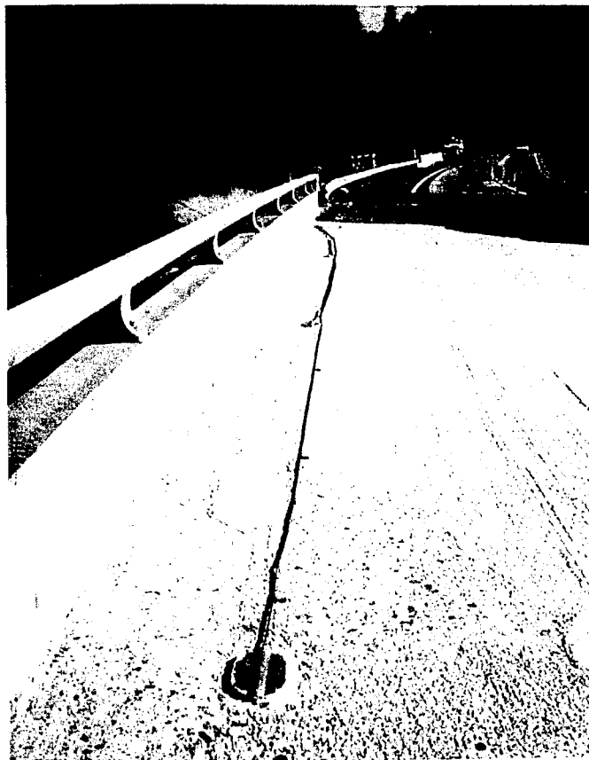
FIGURE 5.3-C Cast Iron Primary Anodes in Place, Coke Breeze CP System, Upper Salt Creek UC (Left)
