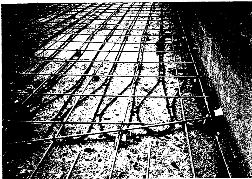
FIGURE 5.5-F Epoxy Coated Reinforcing Steel Over Raychem “Ferex 100” Distribution Anode, Upper Salt Creek UC (Right)
