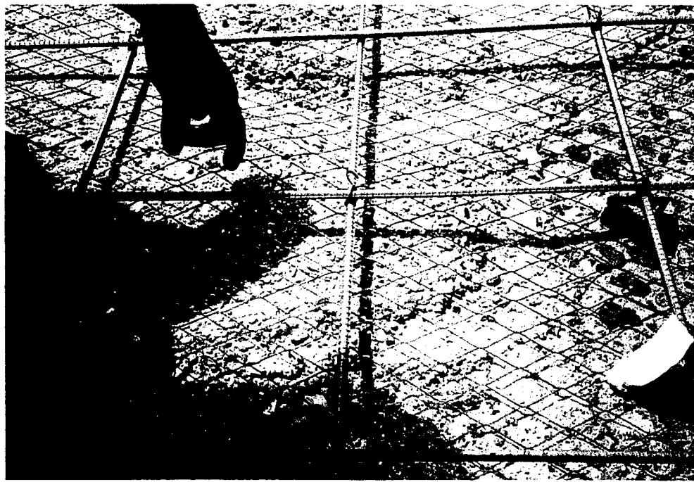
FIGURE 5.6-D Typical Placement of Reinforcing Steel Mat Over Eltech “Elgard 210” Distribution Anode Mesh, Upper Salt Creek UC (Right)
