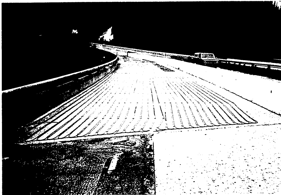
FIGURE 5.5-B Primary Anode Placement, Raychem "Ferex 100" CP System, Upper Salt Creek UC (Right)
