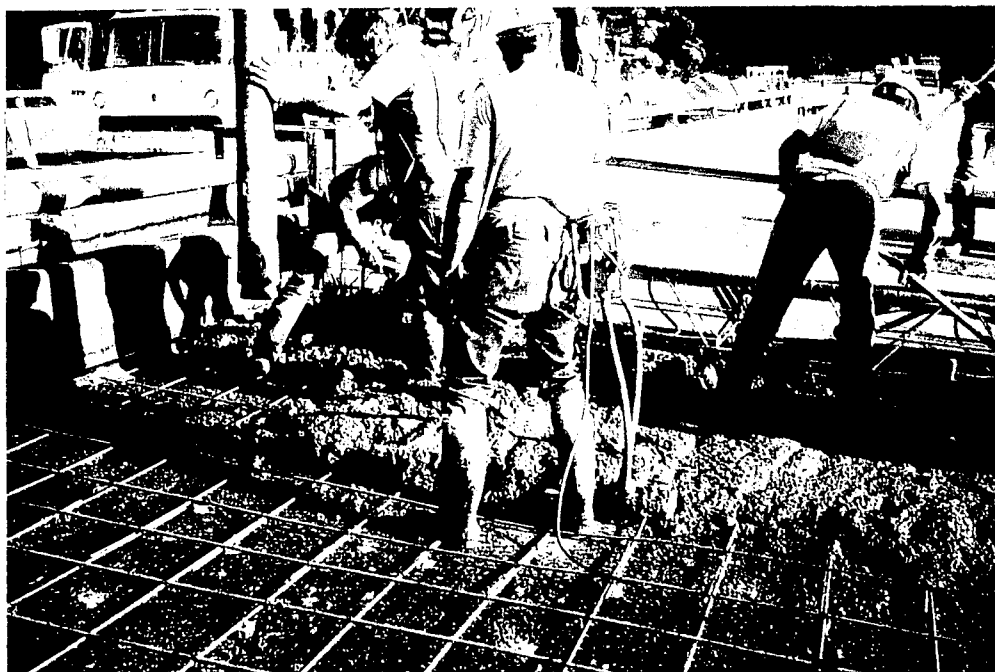
FIGURE 5.5-G Placing Low Slump Concrete Over Raychem and Eltech CP Systems, Upper Salt Creek UC (Right)
