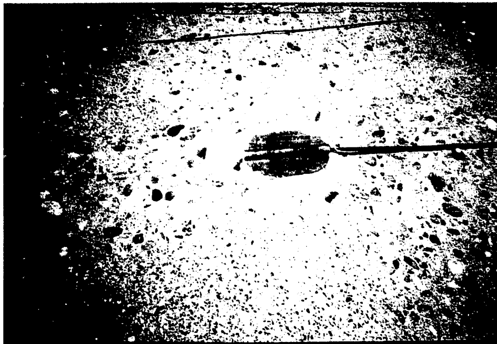
FIGURE 5.3-B Cast Iron Primary Anode Epoxied to Deck, Coke Breeze CP System, Upper Salt Creek UC (Left)
