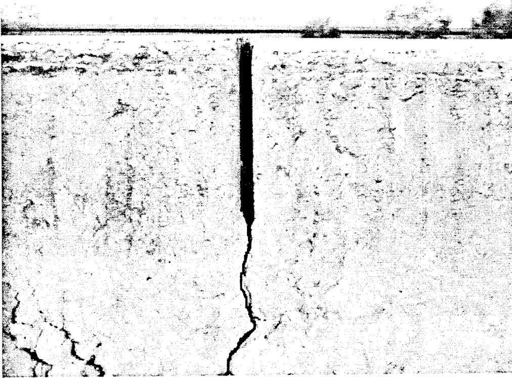
Figure 47a: Photo of Joint 1. Joint crack is enhanced for easier viewing.
