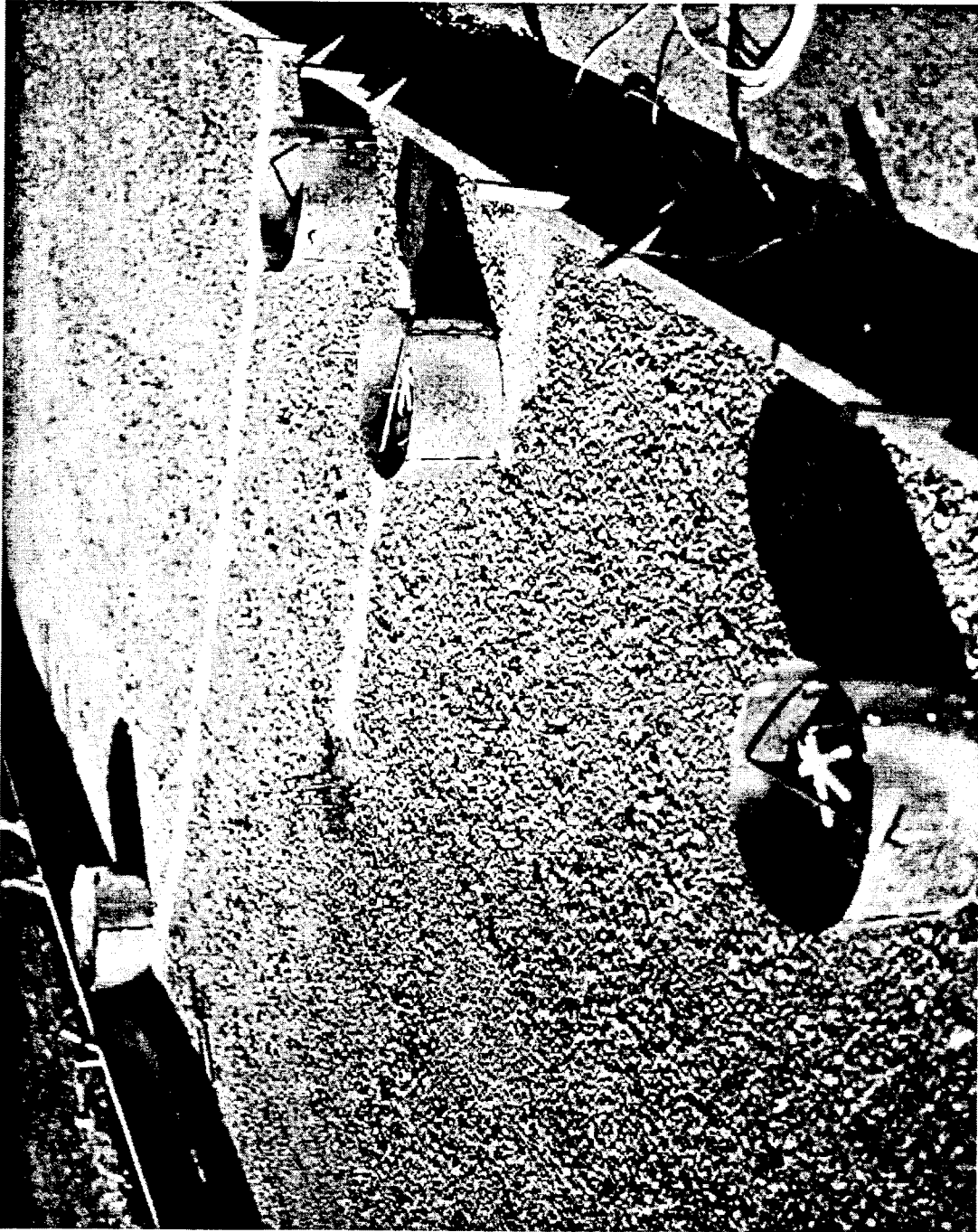
Figure 22. Sheet metal boxes are used to protect strain gages from flow of fresh concrete.
