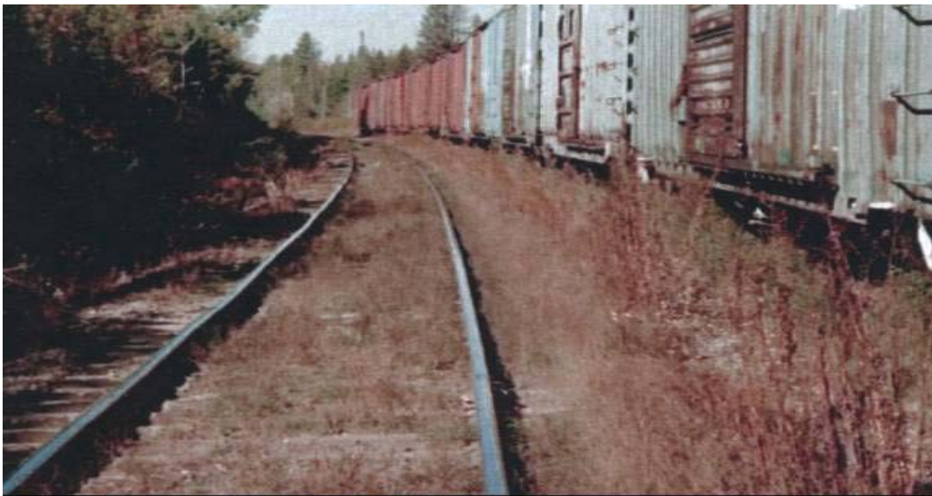
Figure 10 Typical “intensive treatment” track condition.
