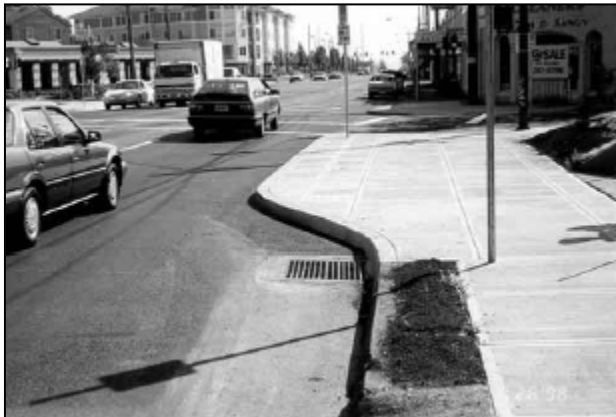
Figure 1. Example of Bus Bulb (Source: TCRP 65).
