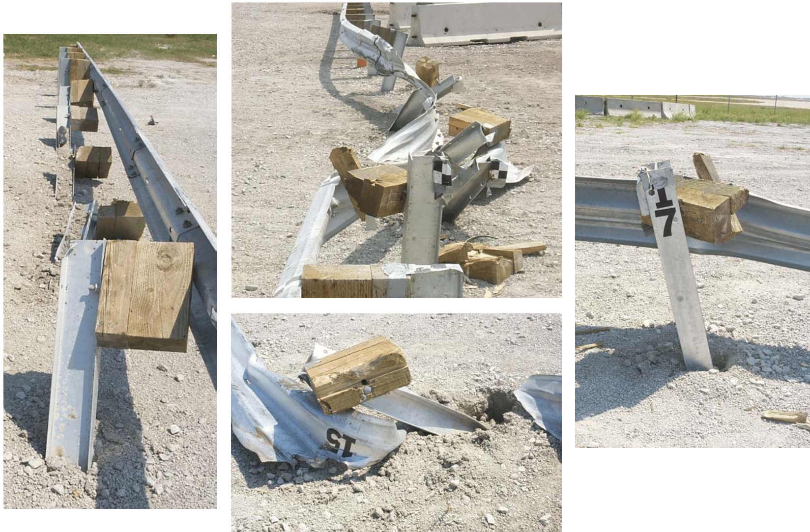
Figure 66. System Damage, Test NPG-2
