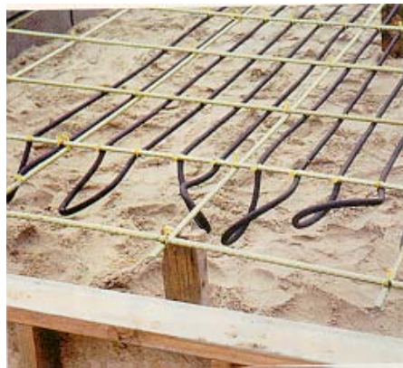
Figure 2.6 Deck heating system on approaches of a pedestrian overpass in Lincoln, Nebraska, 1993
