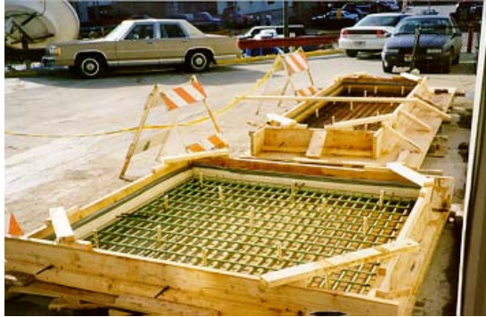
Figure 5-1(a) Slabs ready for casting the conventional concrete layer
