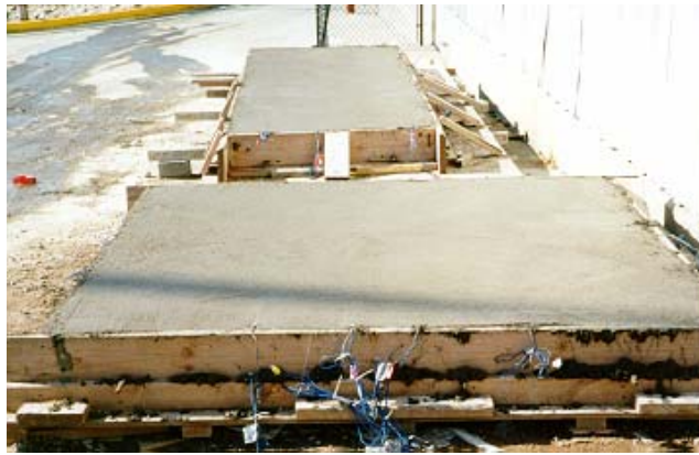
Figure 5-6 Slabs after finishing
