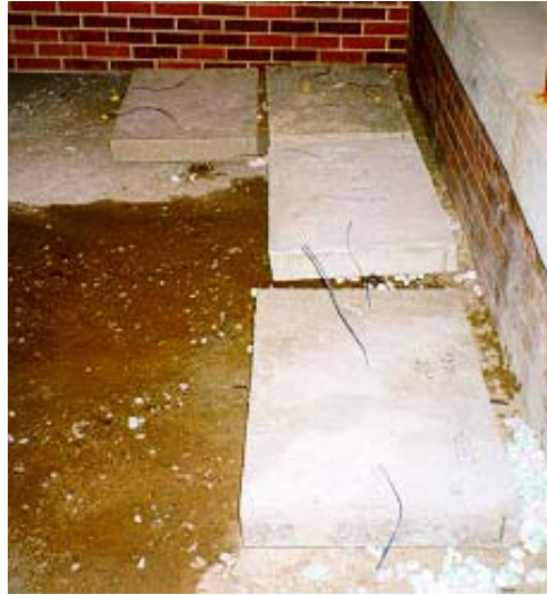
Figure 3-15(b) 3 ft x 2 ft x 3.5 in. slabs
