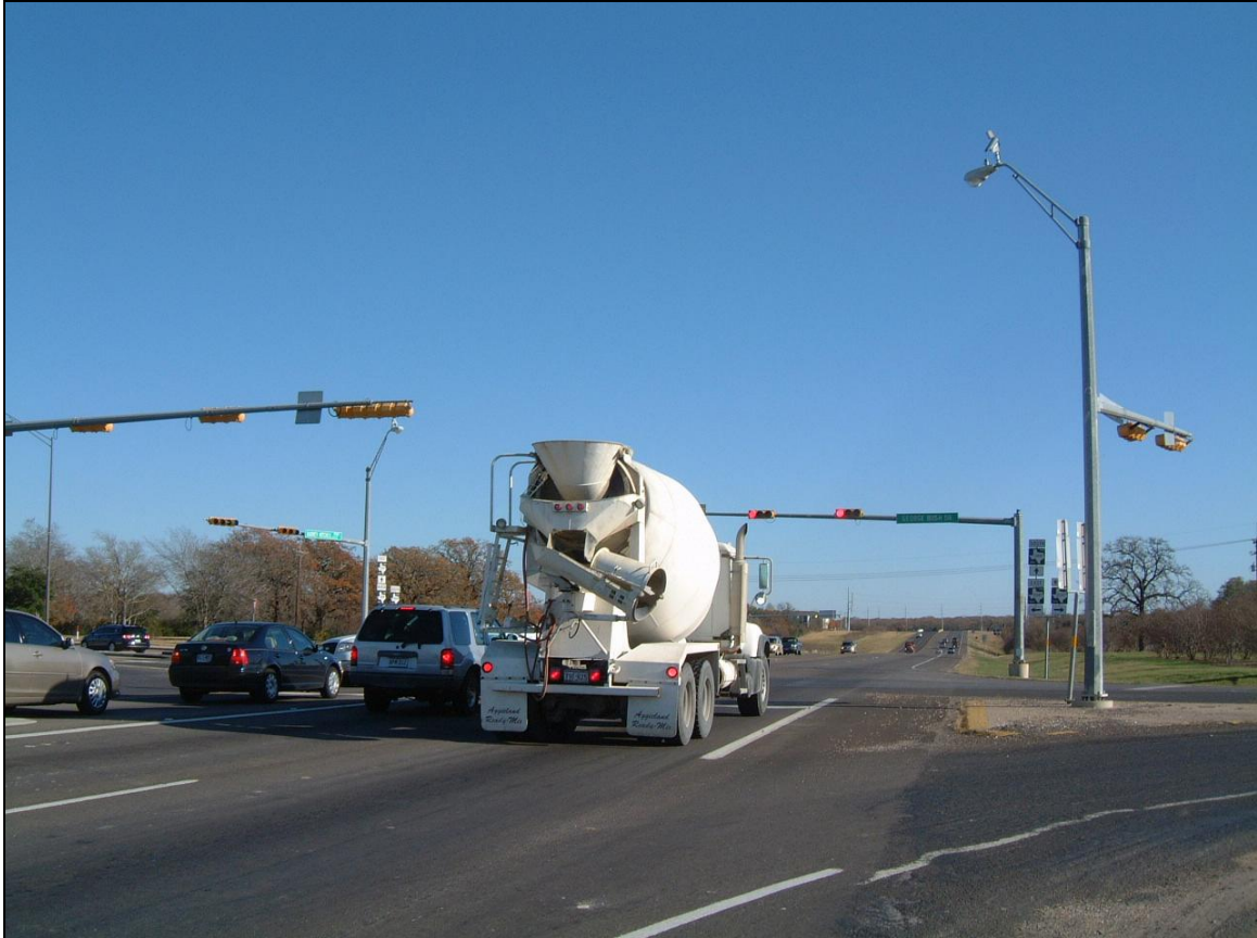
Figure 3. F.M. 2818/George Bush Drive Intersection.
