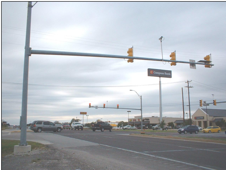
Figure 4. Ft. Worth District VIVDS High-Speed Intersection Installation.
