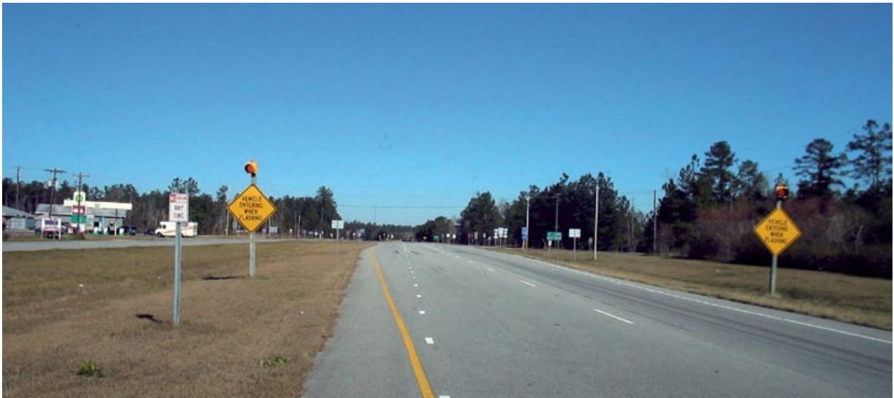
Figure 2: Through Vehicle Activated Warning Sign System in North Carolina
