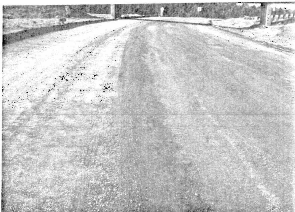
FINISHED BASE GRAVEL
