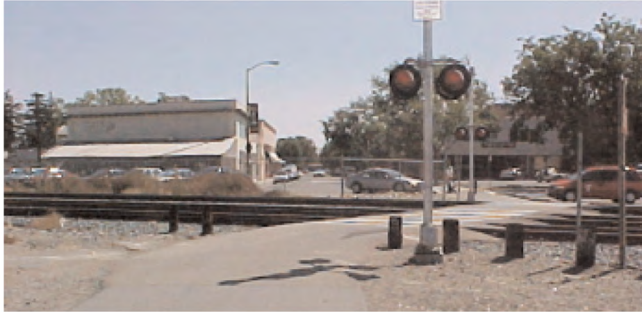
At-grade crossing. Dixon, CA
