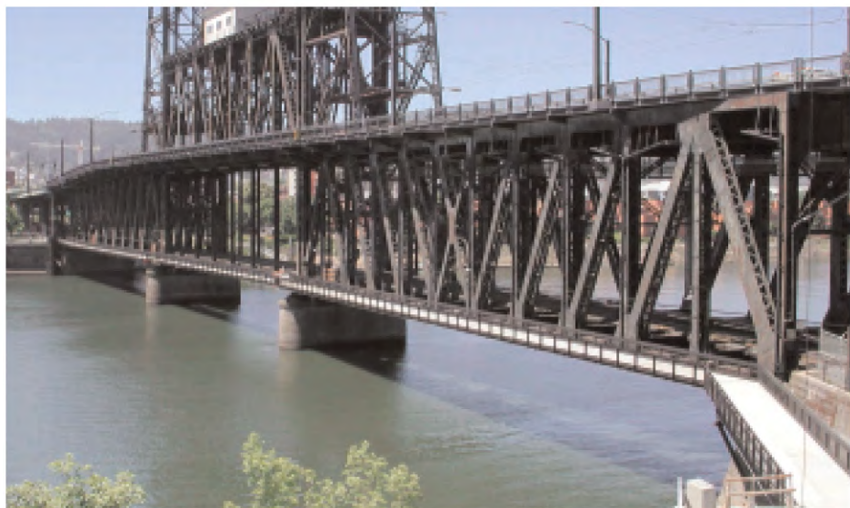
Steel Bridge Riverwalk. Portland, OR
