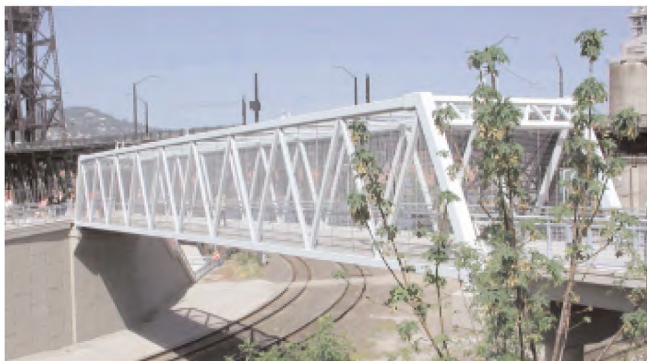
Bridge over Union Pacific tracks. Portland, OR
