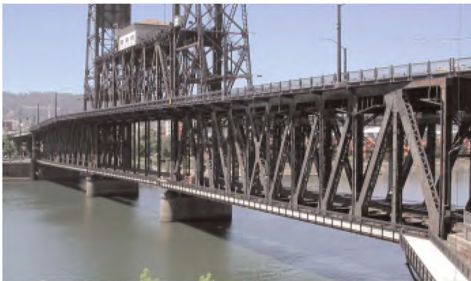
Steel Bridge Riverwalk. Portland, OR
