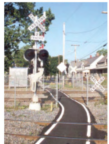
Dual track grade crossing. Burlington, VT
