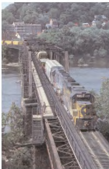
Harpers Ferry Bridge. Harpers Ferry, VA
