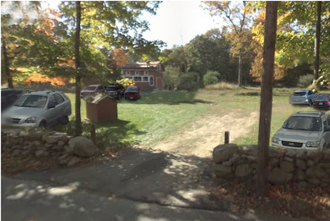
Figure 27 View 1 of Chicken House from path with parked cars Source: U.S. DOT staff
