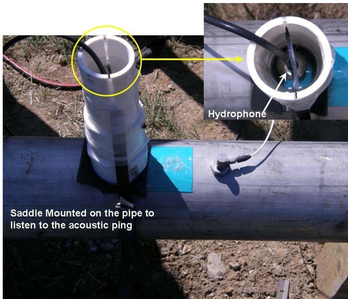
100ft Pipeline setup at DNV outdoors
