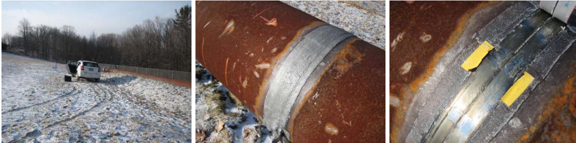
Figure 38. Photos from the 2 nd SHM testing: scenery of the test bed (left), installed sensors on 20-inch bare pipe (middle), and the iron-cobalt strips exposed after the wax tape and MsS ribbon coils were removed (right)
