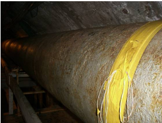
MsS installed on 26" gas pipeline in the Astoria Tunnel
