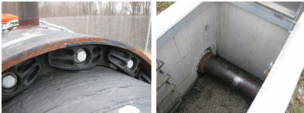
Figure 1. Link seal at the edge of casing (left) and vaulted access to the buried test pipe (right)
