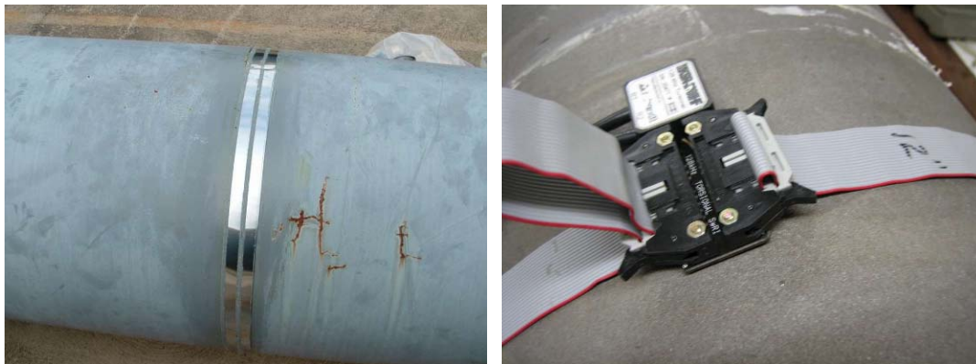
Figure 2. Photo of thin strips bonded around a pipe (left) and the MsS coil placed over the strip (right)
