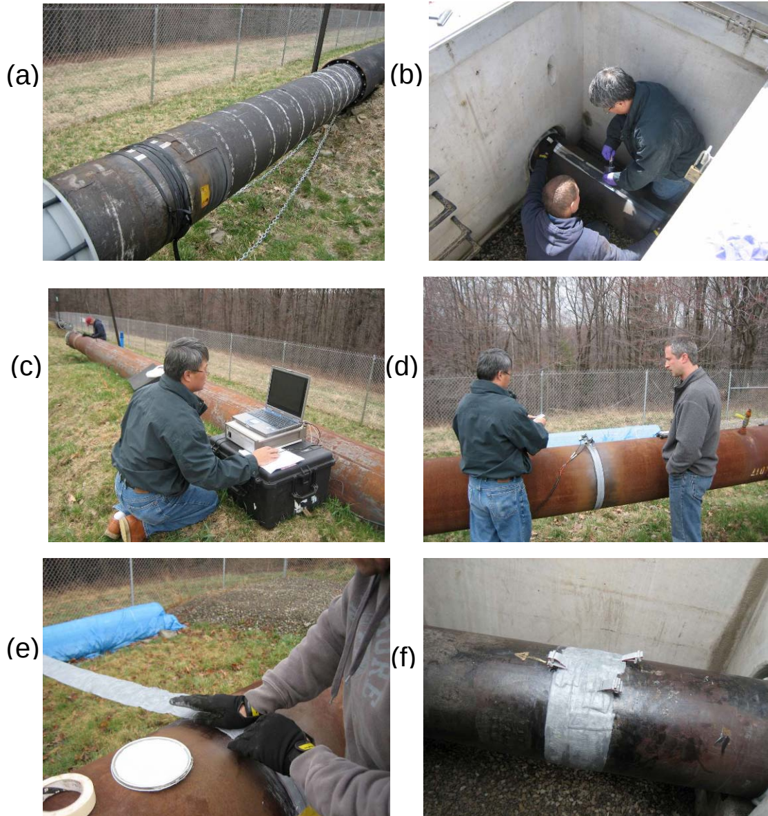
Figure 37. Photos of MsS testing at the NYSEARCH/NGA test bed facility: (a) rubber strap wrapped over the magnetostrictive strips bonded around the 16-inch-OD TGF-3-coated pipeline, (b) applying epoxy on the magnetostrictive strips for bonding to the 12-inch-OD CTE steel pipeline, (c) MsS system during data acquisition from the 20-inch-OD bare steel pipeline, (d) MsS ribbon coils placed over the magnetostrictive strips for testing, (e) wax tape applied over the MsS ribbon coils for protection from environment for long-term monitoring, and (f) MsS ribbon coils installed with protective wax tape on the 12-inch-OD CTE steel pipeline; the exposed ends of the ribbon coils were later wrapped with plastic tape for protection.
