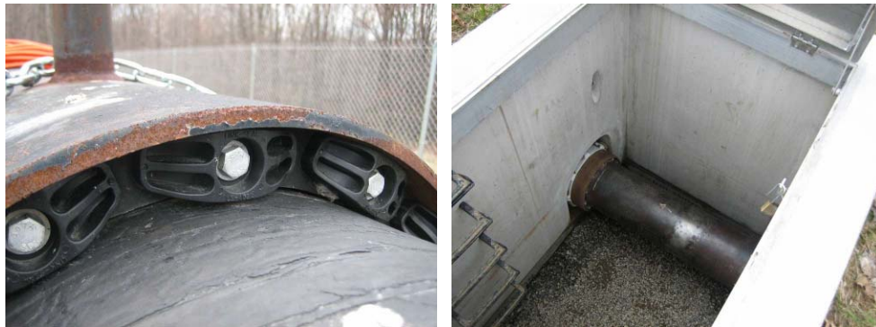
Figure 36. Photos of link joint seal at the edge of casing (left) and vaulted excavation for access to the underground test pipe (right)
