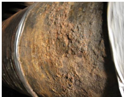
Figure 1. photo of pipe surface at the 1 st test location
