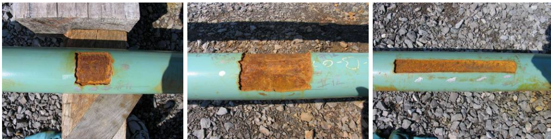
Figure 12. Typical defect induced in the 2nd RG&E mockup: RG&E Defect ID 11
