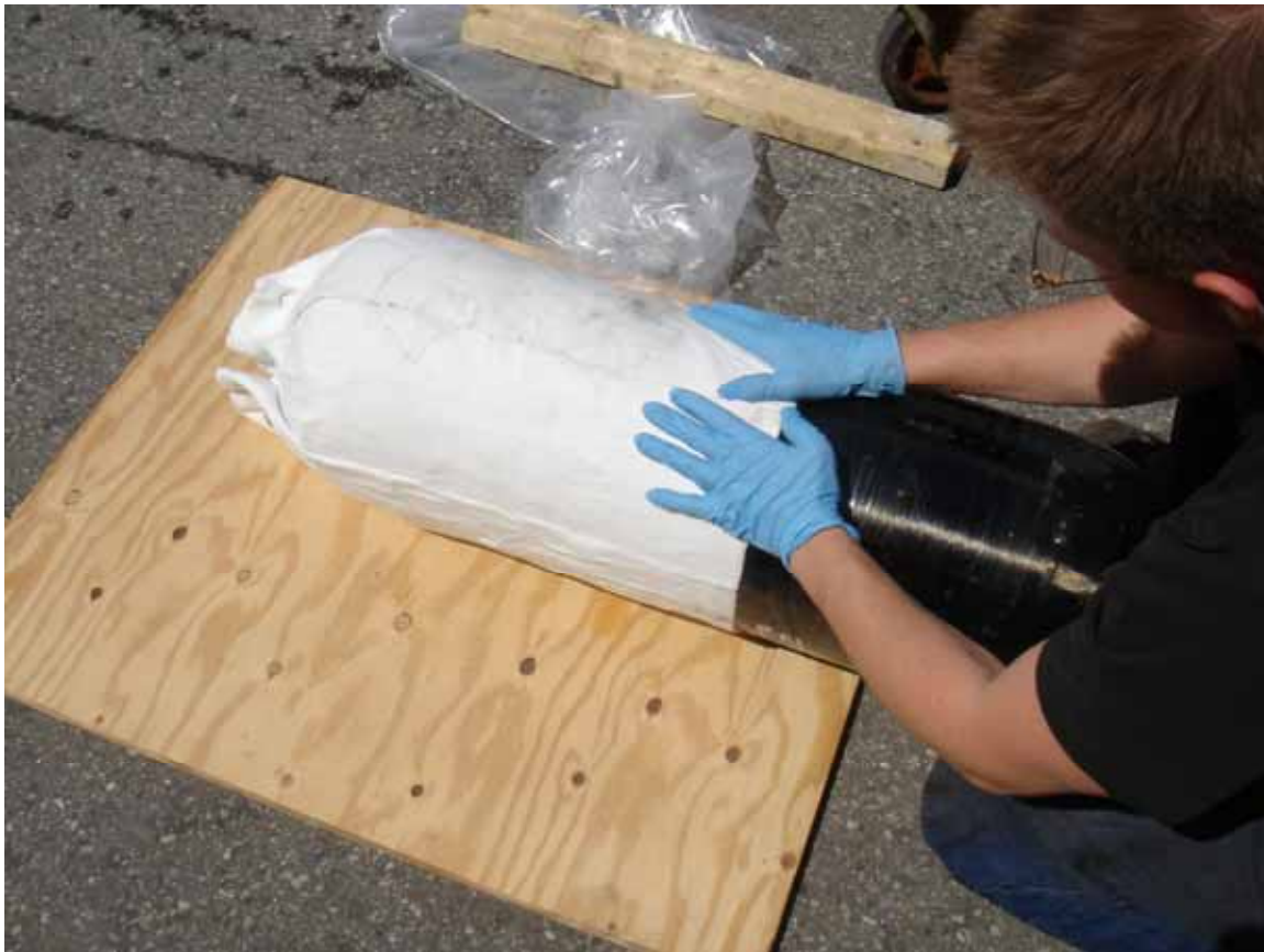
Figure 16 – Application of wet felt wrap to tank
