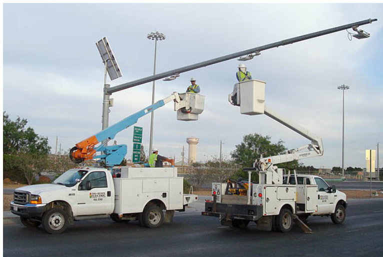
Figure 10. Installing RFID antennae on a mast arm.
