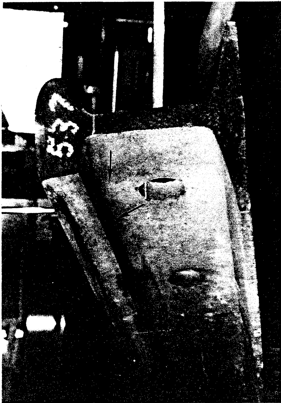
FIGURE 1-7. COMBINED HEAD WEB SEPARATION AND BOLT-HOLE CRACK
