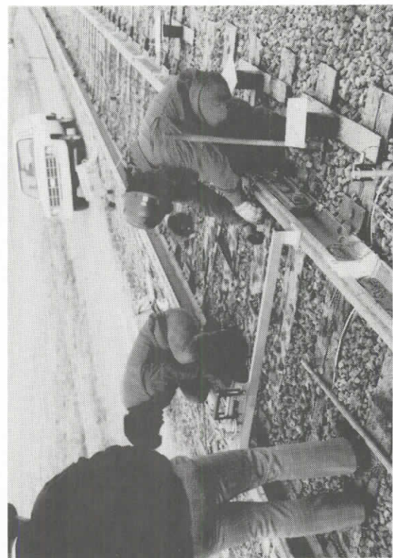
175. TRACK REBUILD - SETTING LOW RAIL TO GAGE USING A COME-ALONG WINCH
