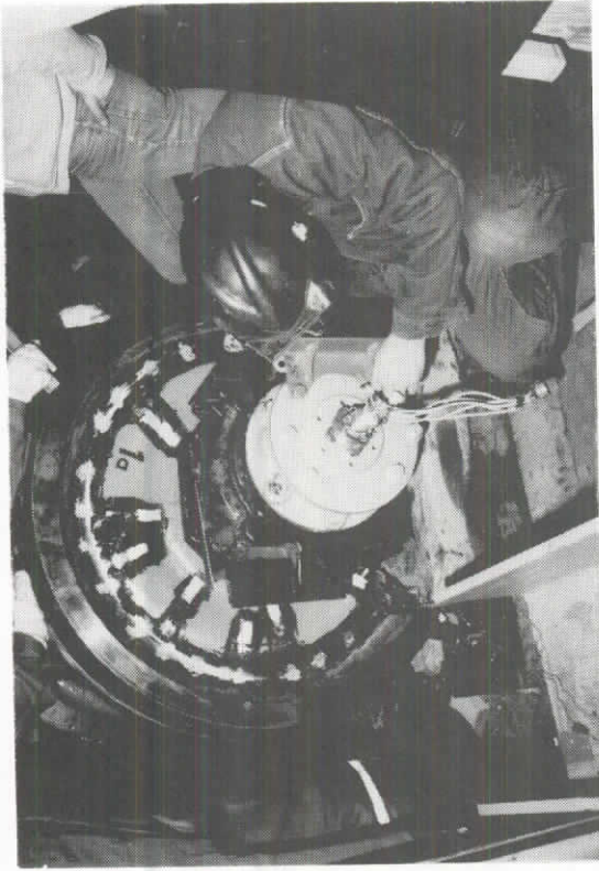
145. REMOVING SLIP RING
