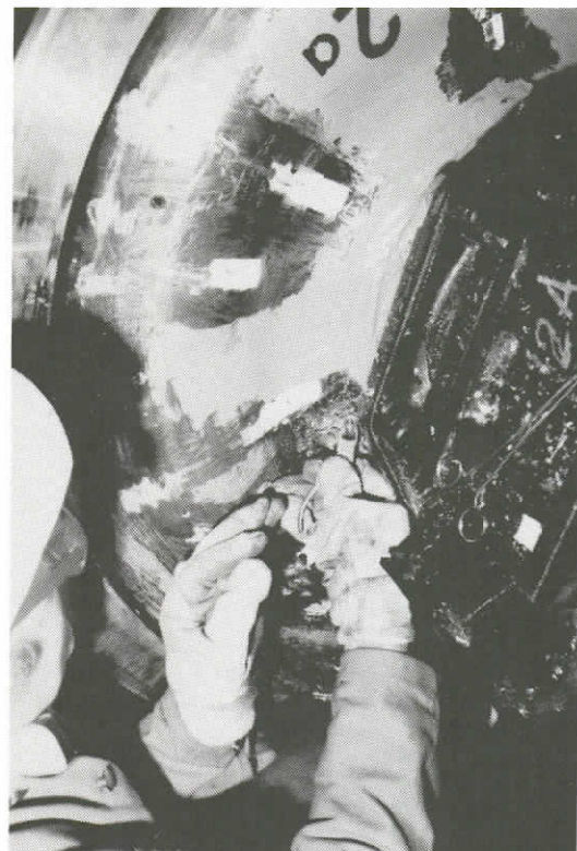
143. REMOVING JUNCTION BOARD
