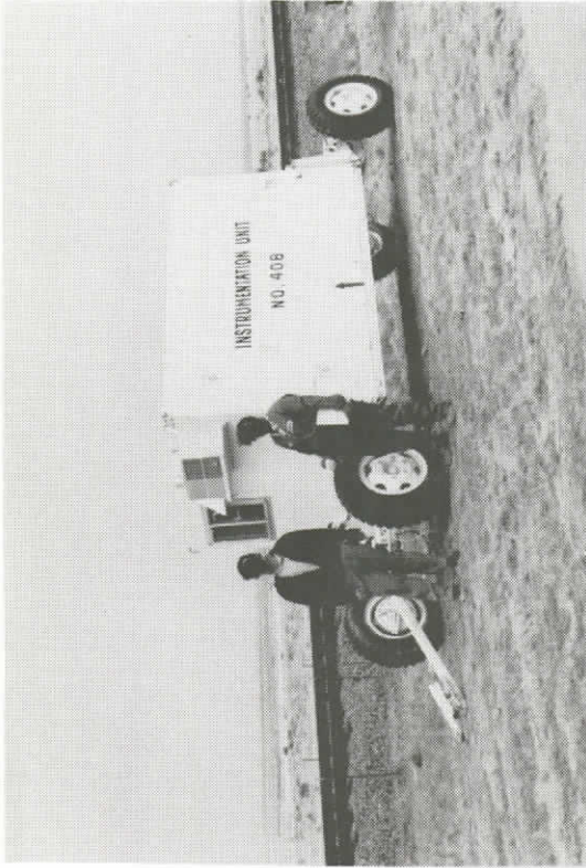
30. TTC DATA COLLECTION UNIT USED IN SECTION 3 FOR MONITORING RAIL DEFLECTIONS
