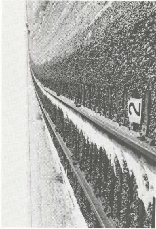
2. SECTION 2 - PIECEWISE LINEAR ALIGNMENT PERTURBATION ON CURVE
