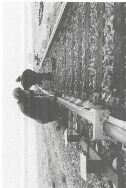
173. TRACK REBUILD - ALIGNING HIGH RAIL BY JACKING AGAINST LOW RAIL AND MEASURING HIGH RAIL OFFSETS FROM 78' STRINGLINE
