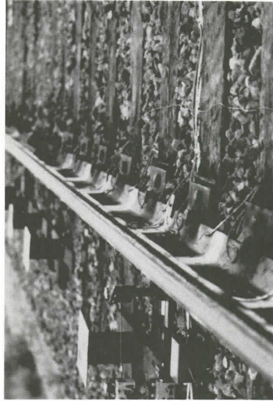
171. SPIKES PULLED DUE TO RAIL ROLL IN SECTION 4
