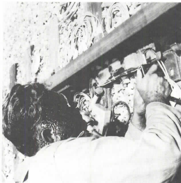
47. TACK WELDING STRAIN GAGE TO RAIL BASE
