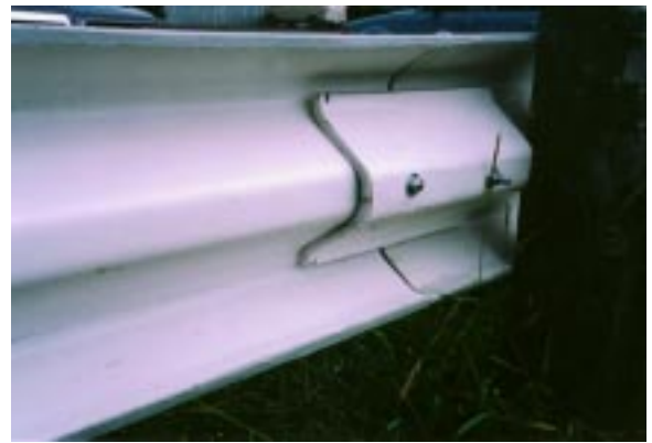
Figure 32. Splicing by cut-out piece of W-beam.
