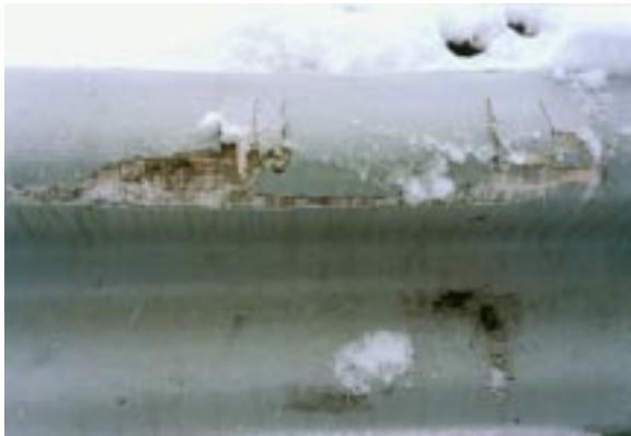
Figure 34. Snow plow abrasion damage to the FRP beam.
