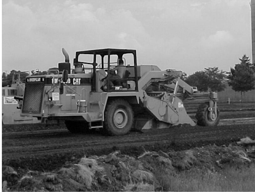
**Figure 1. Pulv mixer used for on-site mixing**
