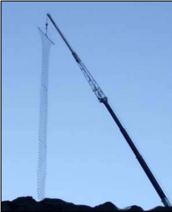
FIGURE 6. Three panel section of Geobrug ring nets with wire mesh; note contraction (necking) of panels.
