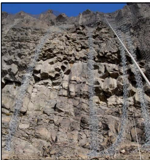
FIGURE 11. View of contracted panels without wire mesh backing.
