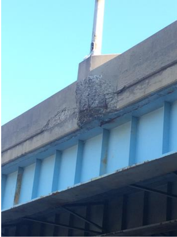
Figure 1 - Typical spall with exposed bar
