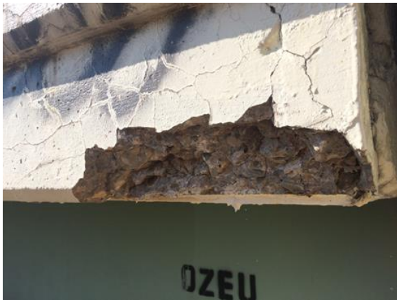
Figure 4 - Map cracking, no indication of corrosion
