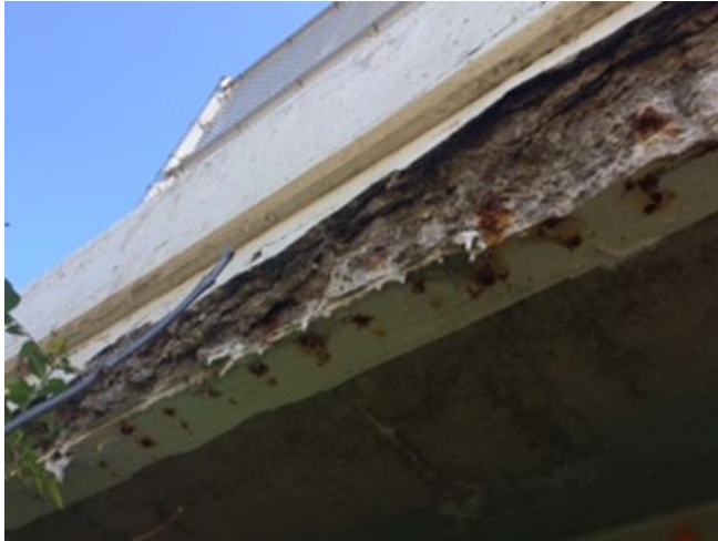
Figure 5 - Severe deterioration with corrosion. The corrosion may have occurred after the concrete was damaged.
