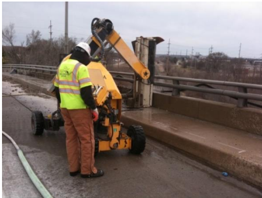
Figure 13: CONJET 327 used on a bridge railing (Photo courtesy of National Hydro, Inc.)
