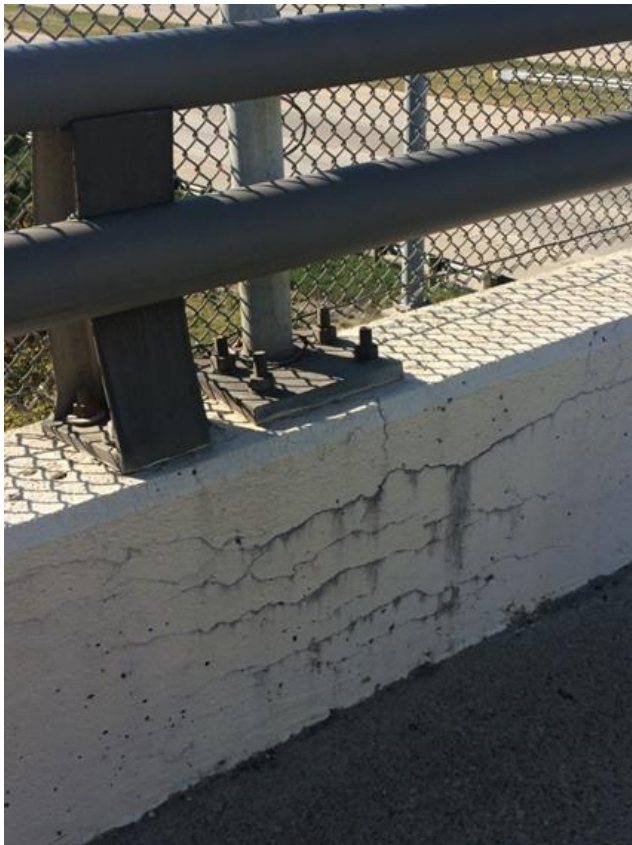
Figure 6 - Cracking on the parapet under a vandal fence support.
