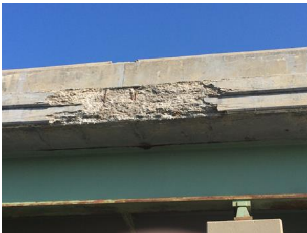
Figure 2 - Spalled concrete with some exposed bar, but with areas with no exposed bar.
