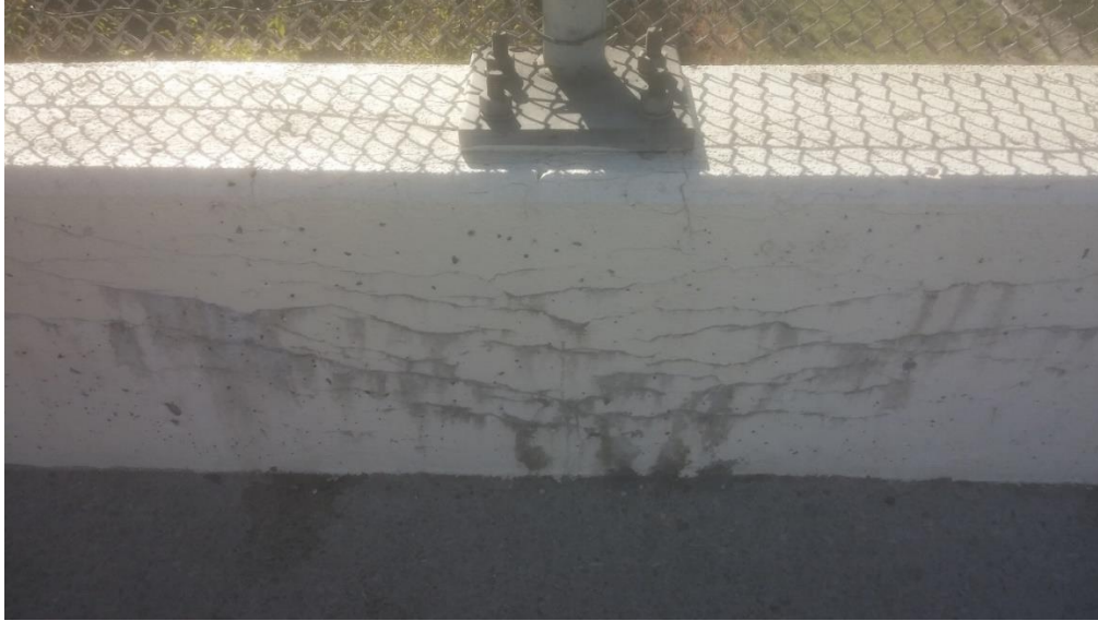
Figure 7 - Cracking on the parapet wall.
