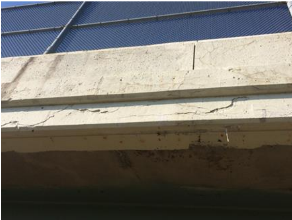
Figure 8 - Cracking on the south face of the bridge.
