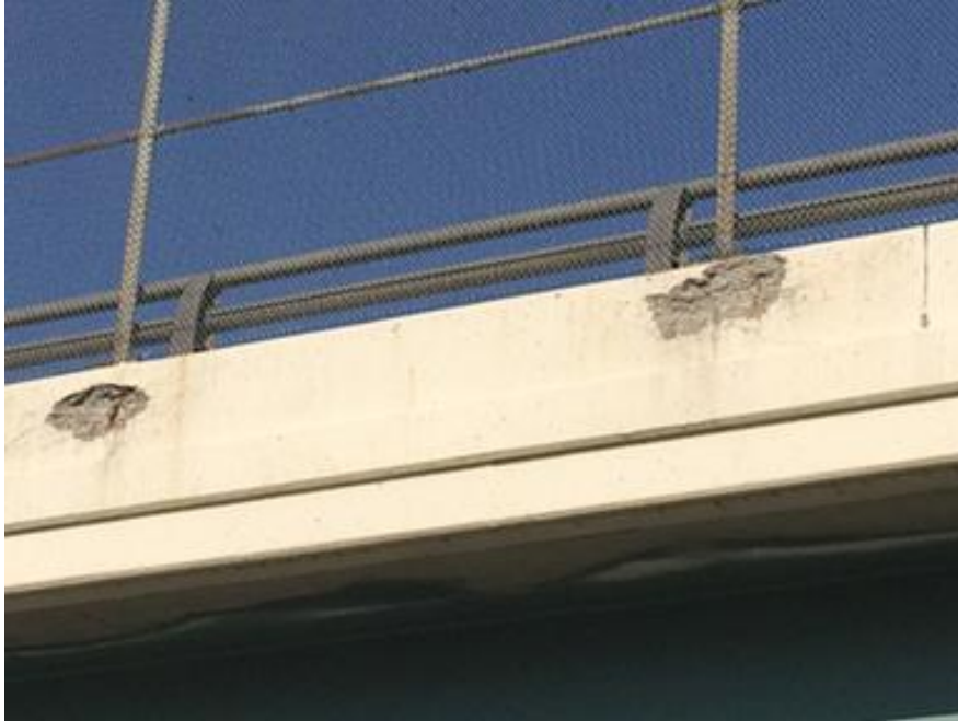
Figure 9 - Spalling on the south face of the bridge.
