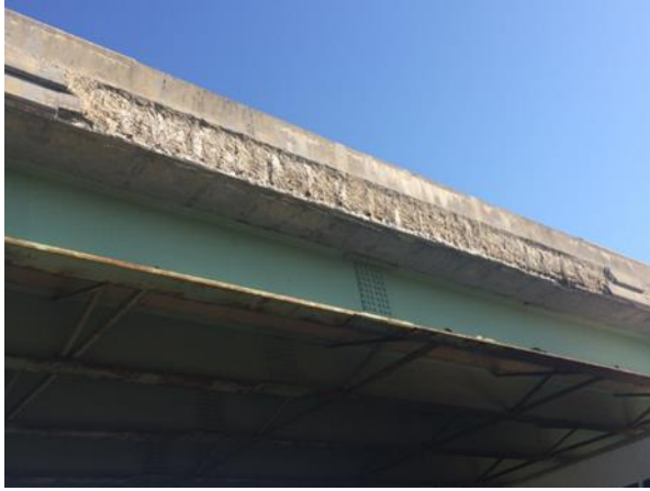
Figure 3 - Damage due to corrosion
