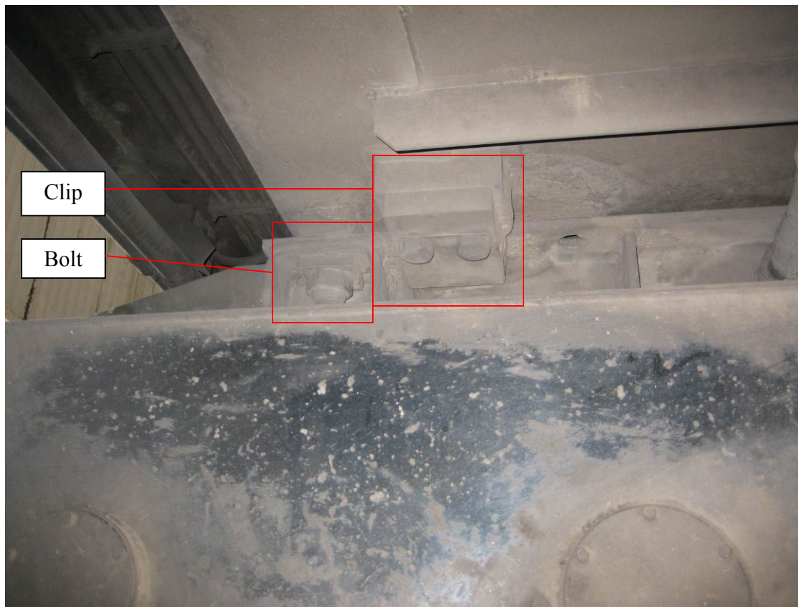
Figure A.3-2. Fuel Tank Attachment to Underframe
