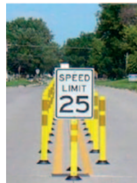
Tubular channelizers in Slater, Iowa
