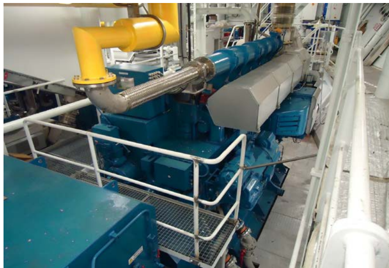
Photo 5: Wärtsilä dual fuel 6L20DF generator set onboard the PSV Viking Princess with double-walled gas supply line in yellow
