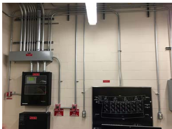
Figure 2-67: Typical U.S. tunnel cable arrangement with conduit (photo opportunity courtesy of Caltrans).
