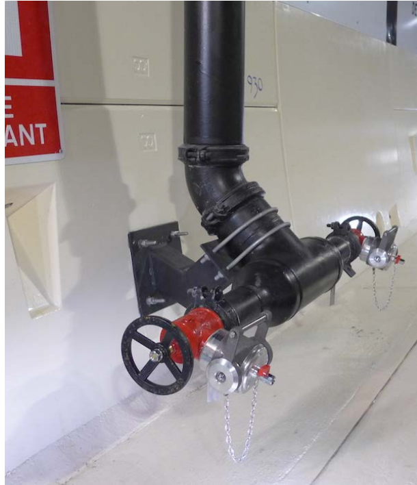
Figure 2-32: Waterview Tunnel fire hose attachment detail.
