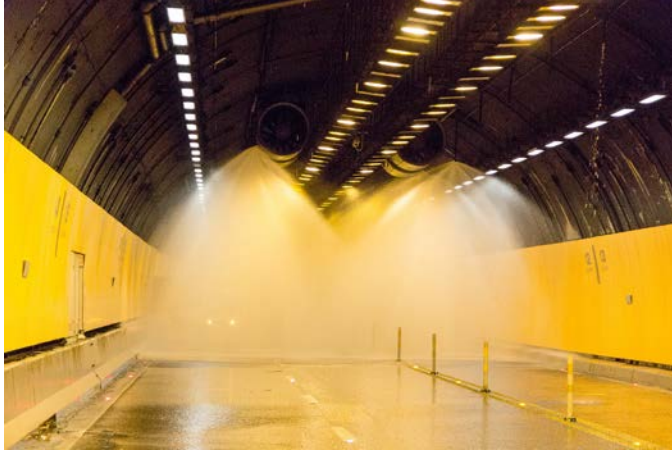
Figure 2-4: FFFS activation in the Terrace Tunnel at water application rate of 0.16 gpm/ft 2 (6.5 mm/min).
