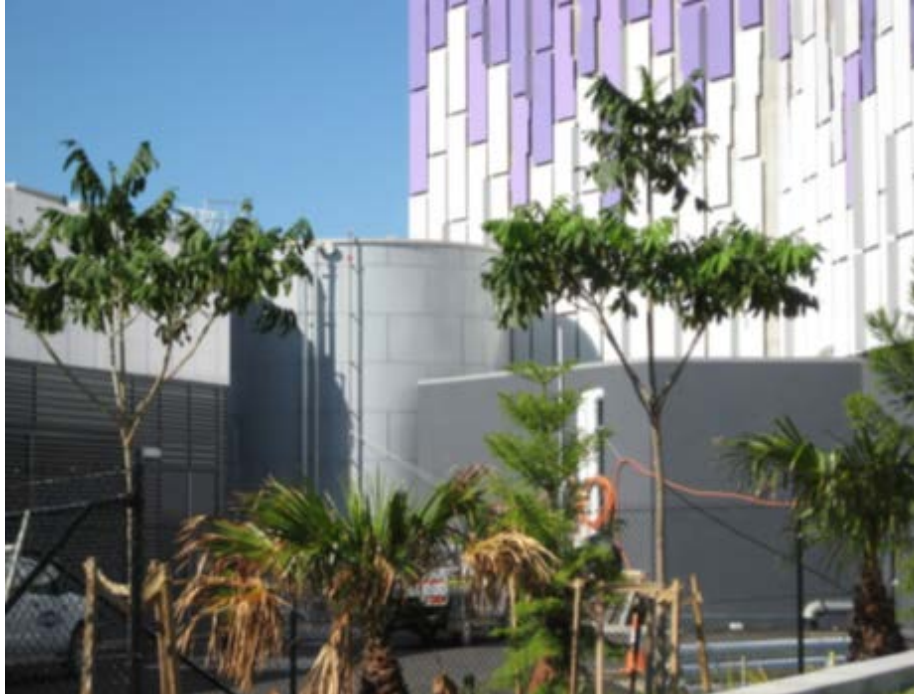
Figure 2-6: Clem7 (Brisbane, Australia) Tunnel water storage tank.
