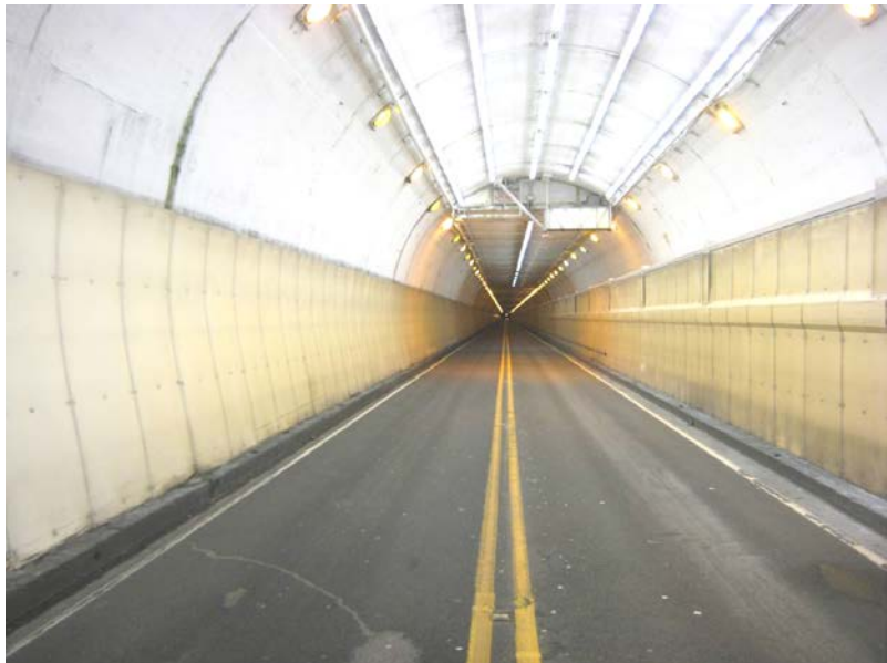
Figure 2-24: Mount Victoria Tunnel prior to rehabilitation.
