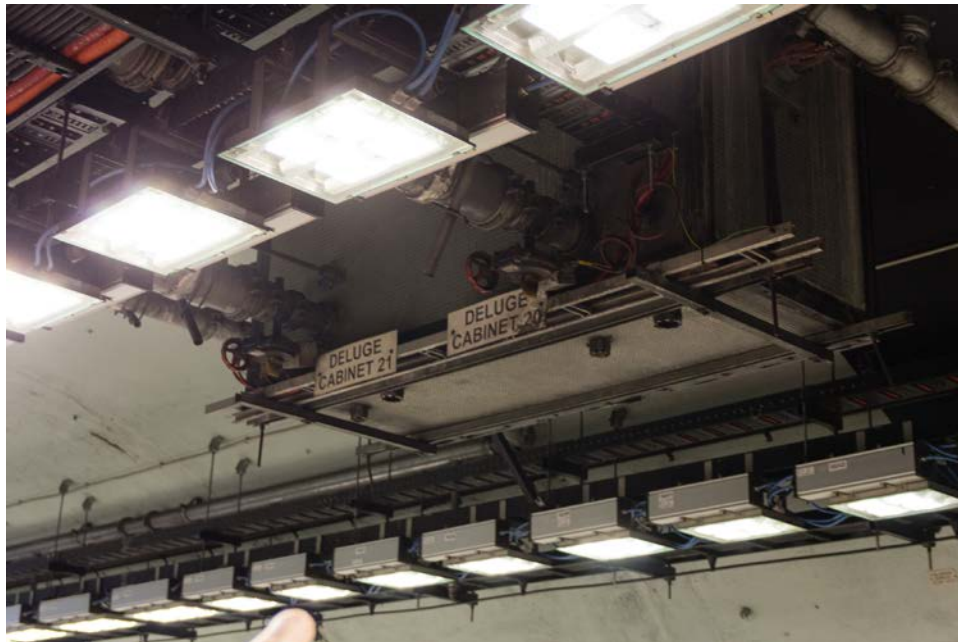
Figure 2-28: Mount Victoria Tunnel close-up of FFFS (deluge) valve in the tunnel apex.
