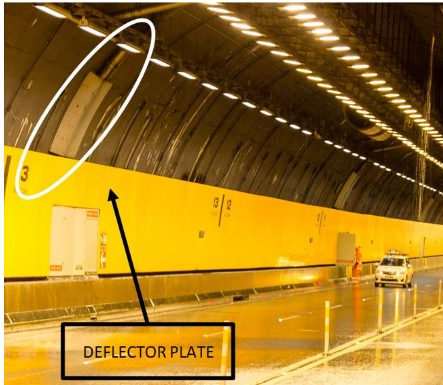
Figure 2-22: Deflector plate installed on the Terrace Tunnel branch main to overcome minor traffic envelope overlap.
