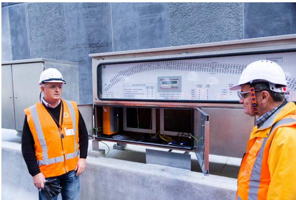
Figure 2-14: Waterview Tunnel fire command post showing screens for incident playback to the response crew.
