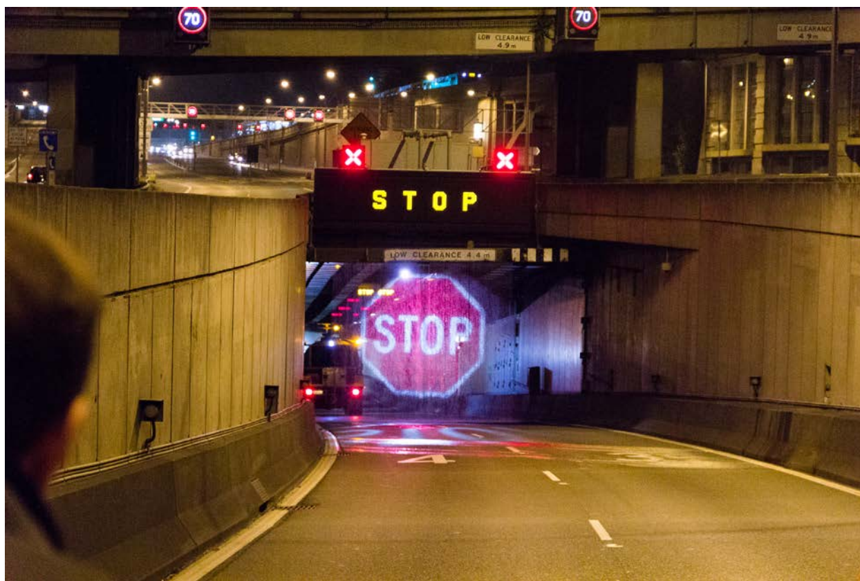
Figure 2-55: Sydney Harbor Tunnel water stop sign projection.
