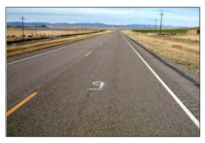
Average transverse cracking per mile (CPM) is low at 37 with a standard deviation of 1. All cracks were sealed. Very little rutting was observed during this evaluation. Estimated average rut is around 2 millimeter on both lanes.
