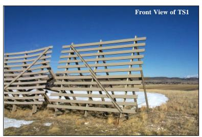
state of Montana. In addition, this experiment was to compare a new design as submitted by the contractor. The modified design deleted the interior rear supports (Test Section 1 [TS1] vs. Test Section 2 [TS2]), as explained in the November 1999 construction report (document address located at the end of this report). As noted in the May 2001 report, TS2 was found collapsed, which was assumed a structural-related failure due to the three rear (sole) supports buckling or snapping in high winds.
