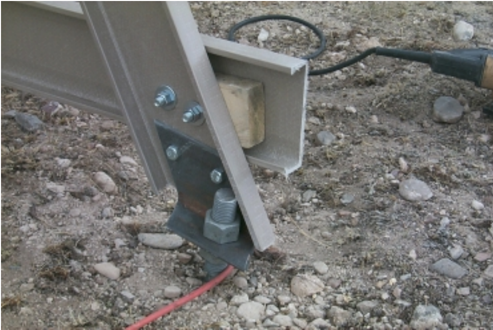
FRP frame attachment to Helical Anchor.
