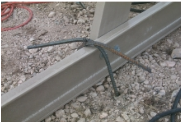
Figure3, Anchor Sill.
