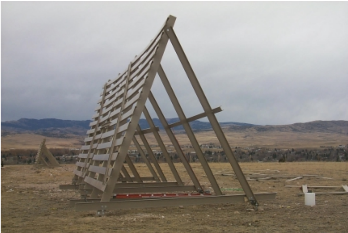
Side view of completed test sections 1 & 2.
