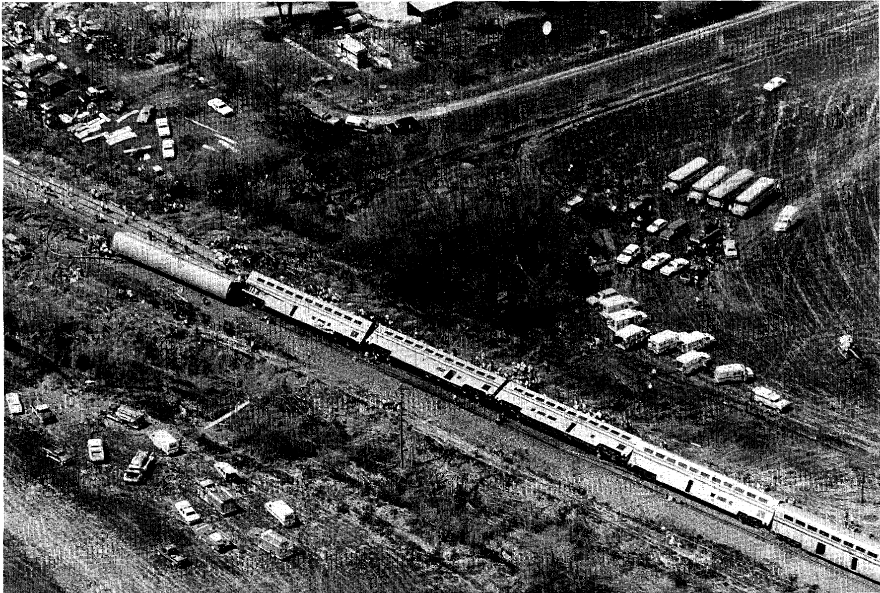
Figure 3.--Accident site photograph.
