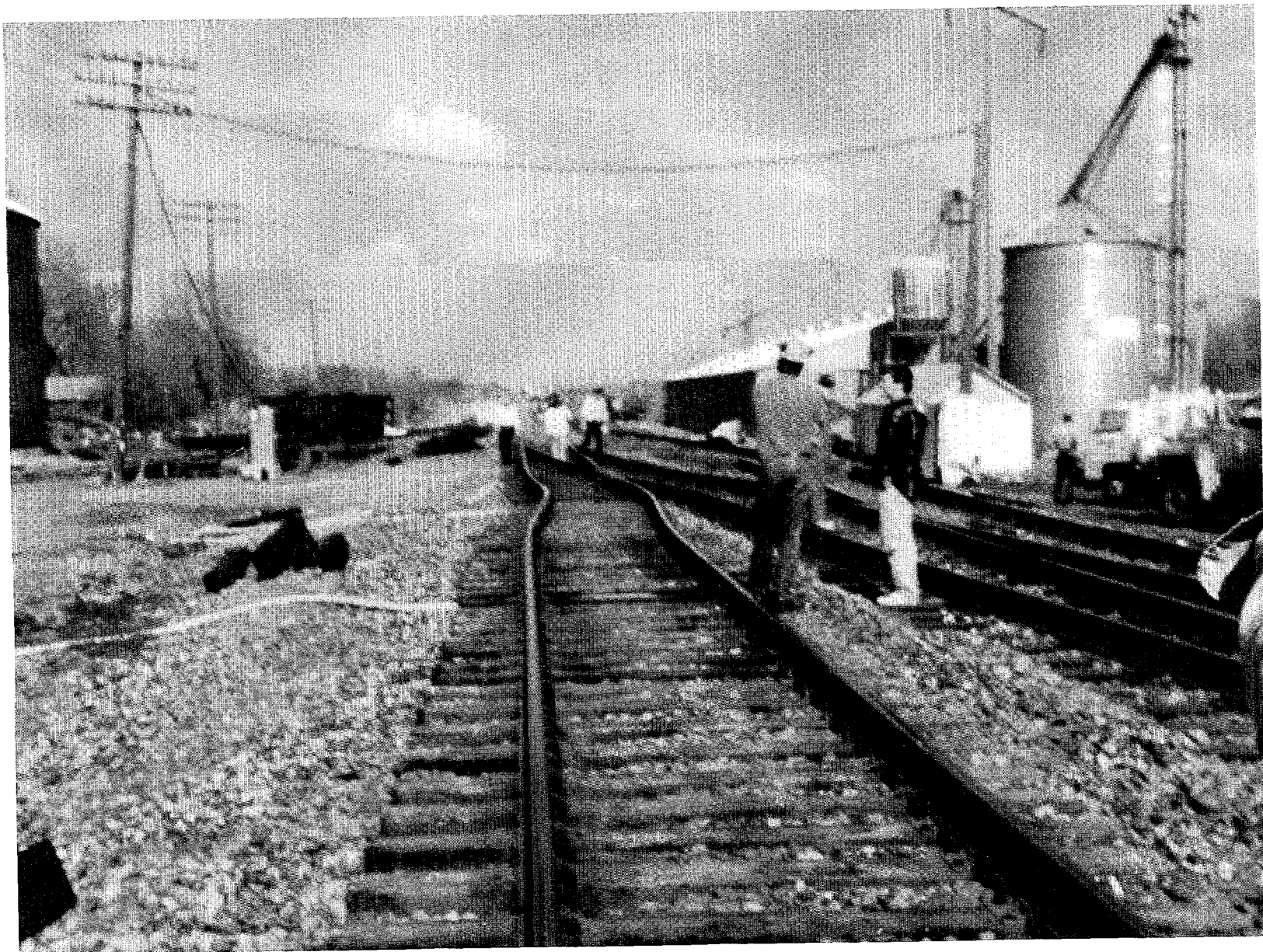
Figure 10.--Westbound mainline track alignment.
