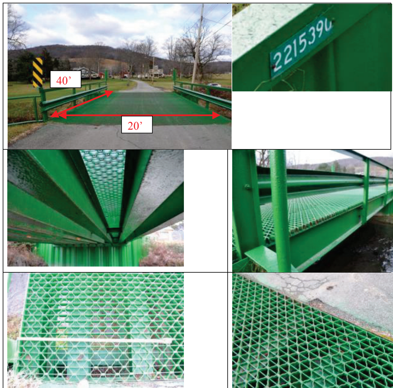
Figure 16. Photos. Existing conditions as of November 2010.
