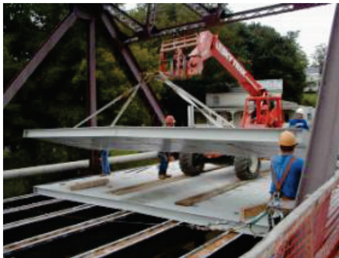
Figure 1. Photo. Typical installation of FRP deck panels on an existing bridge.
