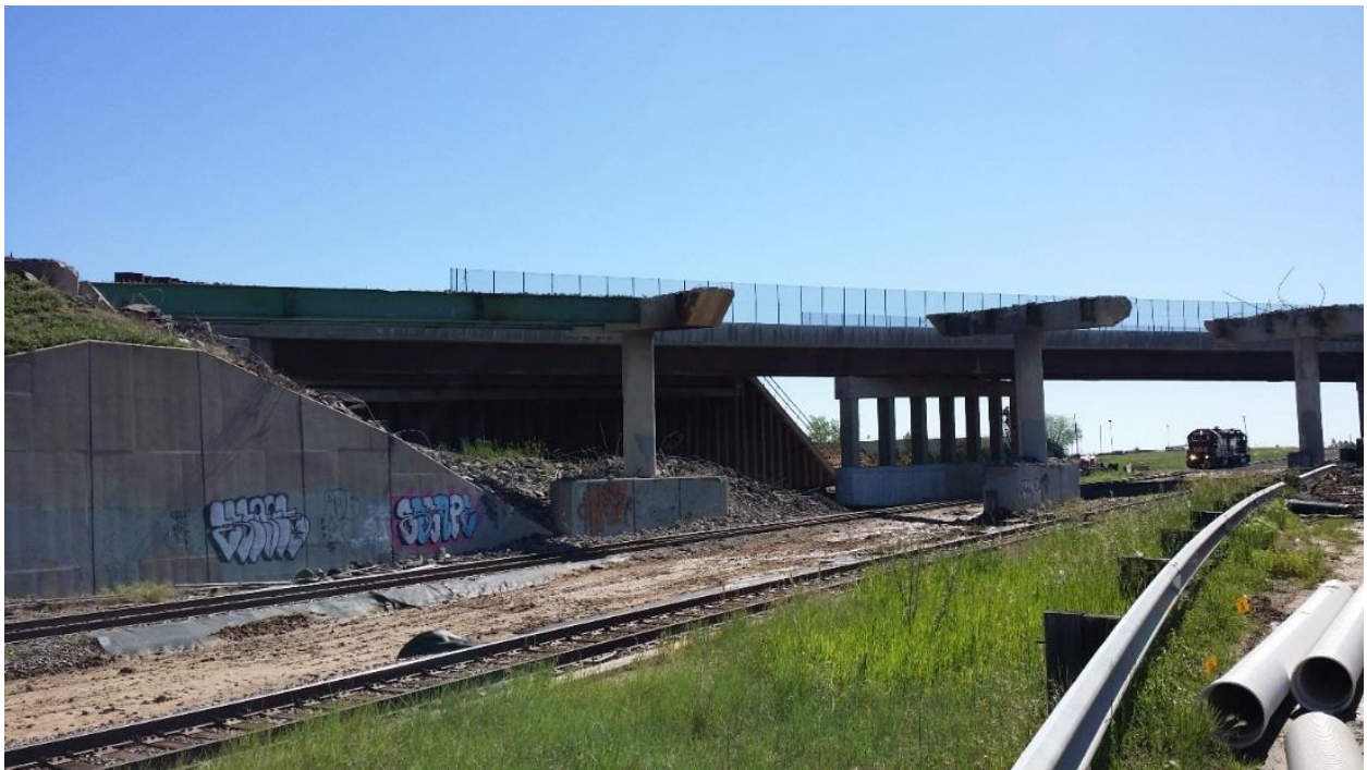
Figure 18. Photo. Old eastbound bridge being demolished, new bridge E-17-AEK in background, June 2015. E-17-AEK is in service at the time of this photograph.
