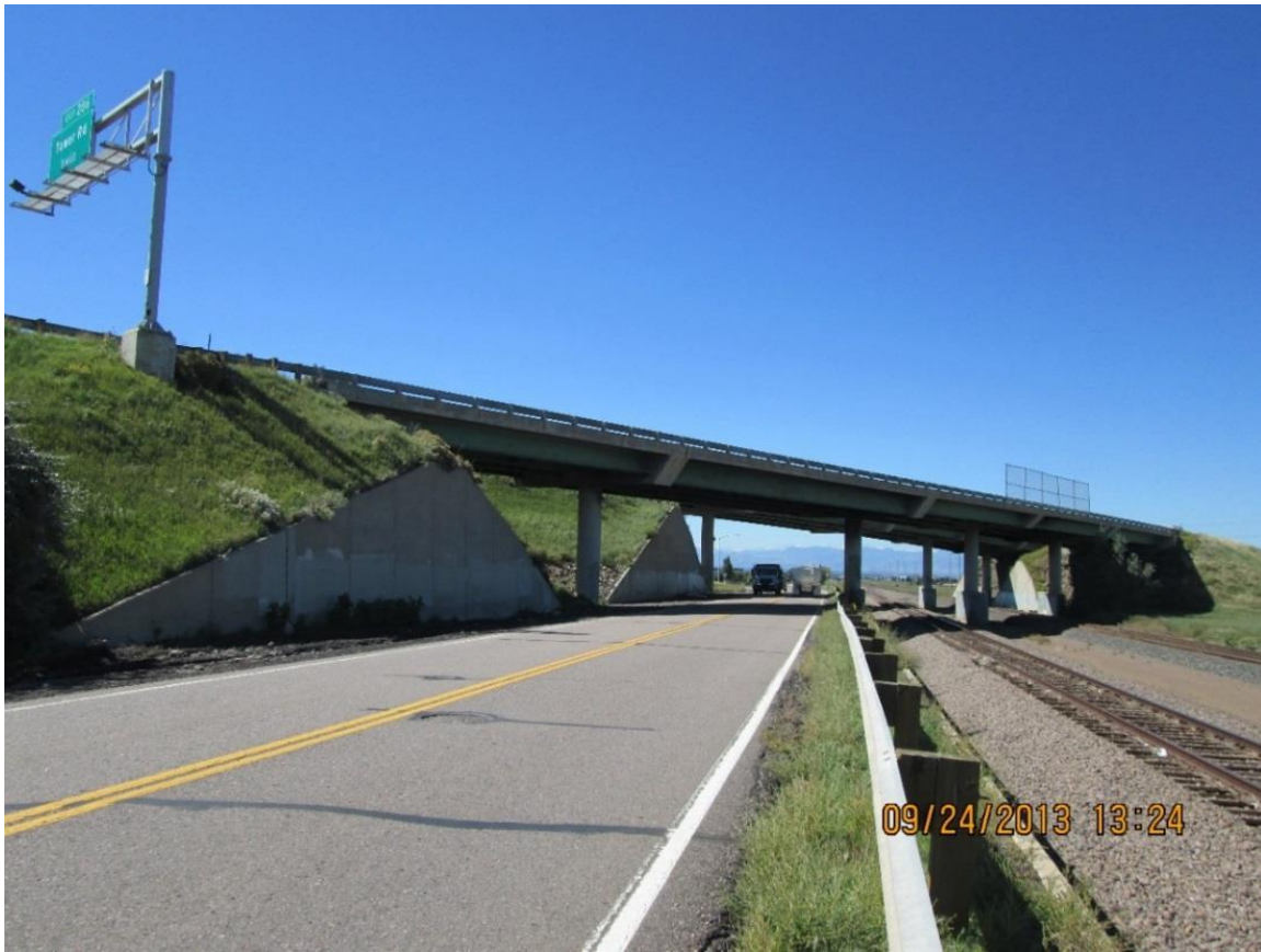
Figure 4. Photo. Bridge E-17-JX (westbound).
