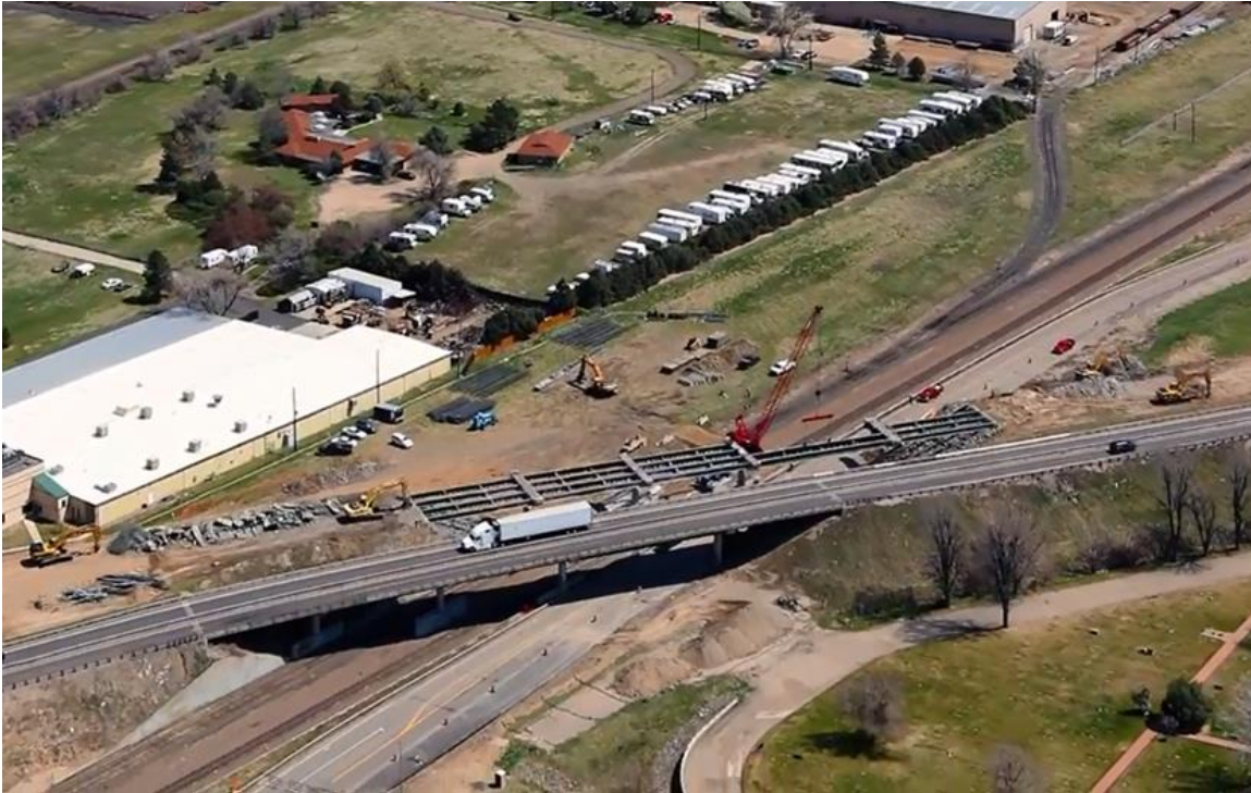
Figure 16. Photo. Steel girder installation for E-17-AEK.
