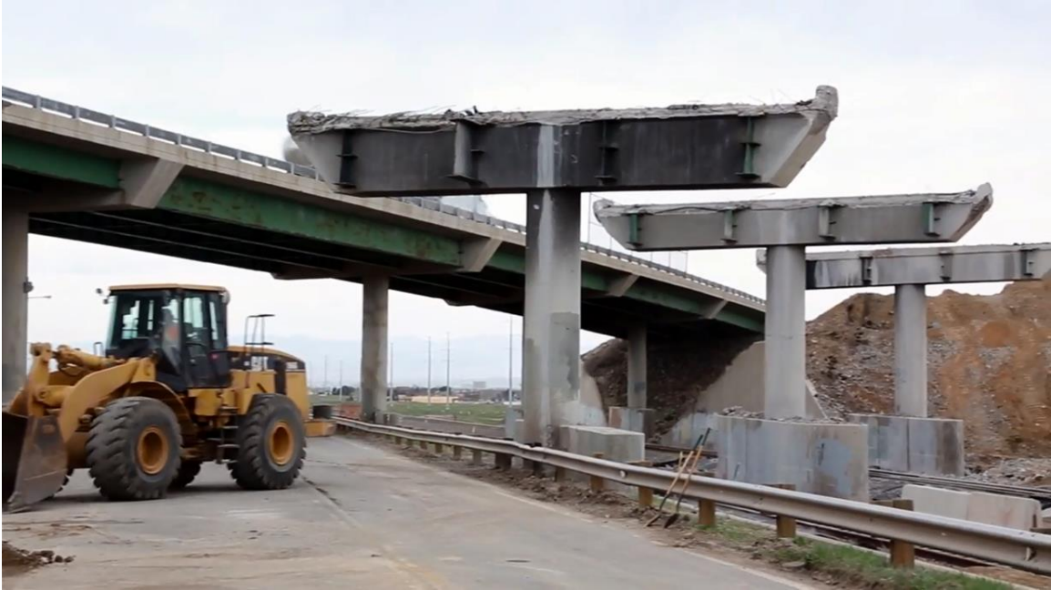
Figure 11. Photo. Old westbound structure, E-17-JX, being demolished.
