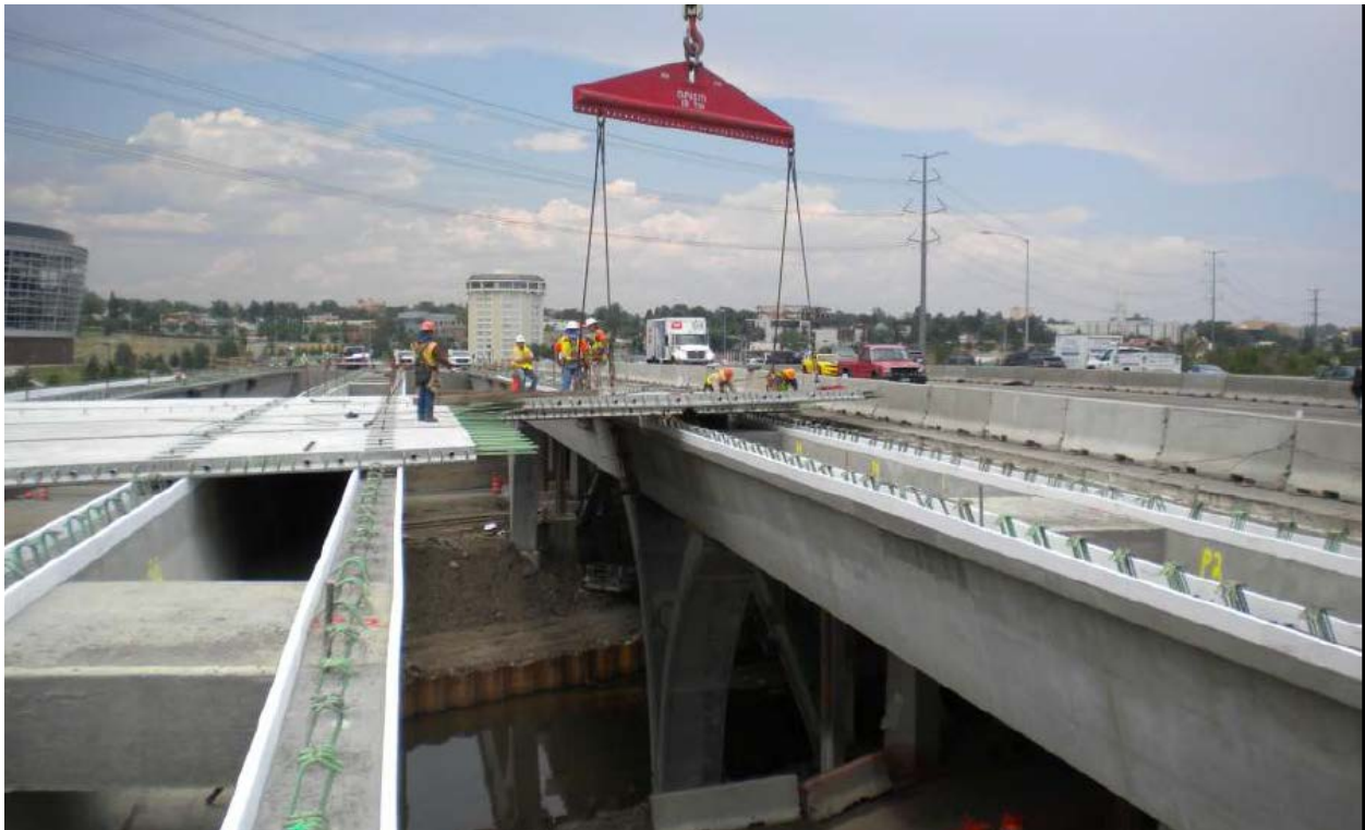
Figure 25. Photo. Panels set with pockets over shear reinforcing in girder top flanges (courtesy: Colorado DOT).
