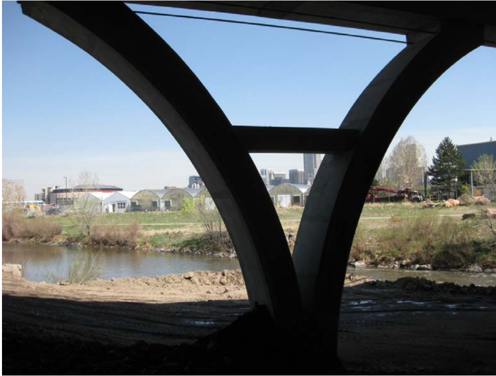
Figure 15. Photo. Arch shaft pier (courtesy: Colorado DOT).
