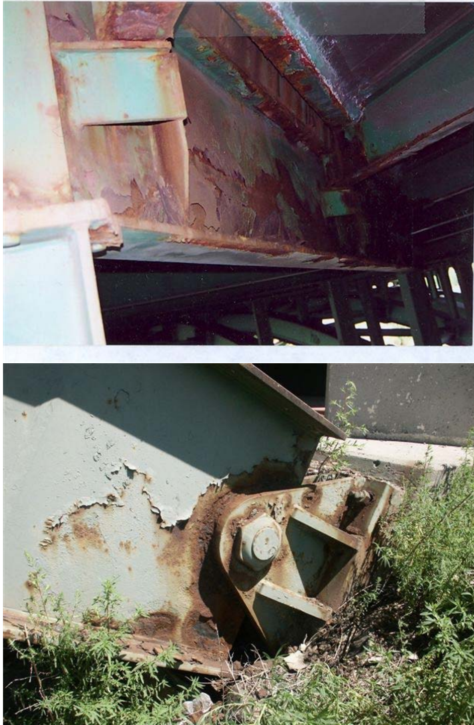
Figure 5. Photos. Deterioration of original structure (courtesy: Colorado DOT).
