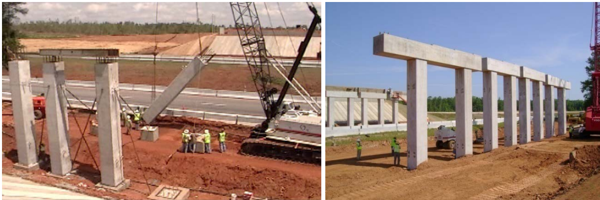
Figure 2. Placement of precast columns.
