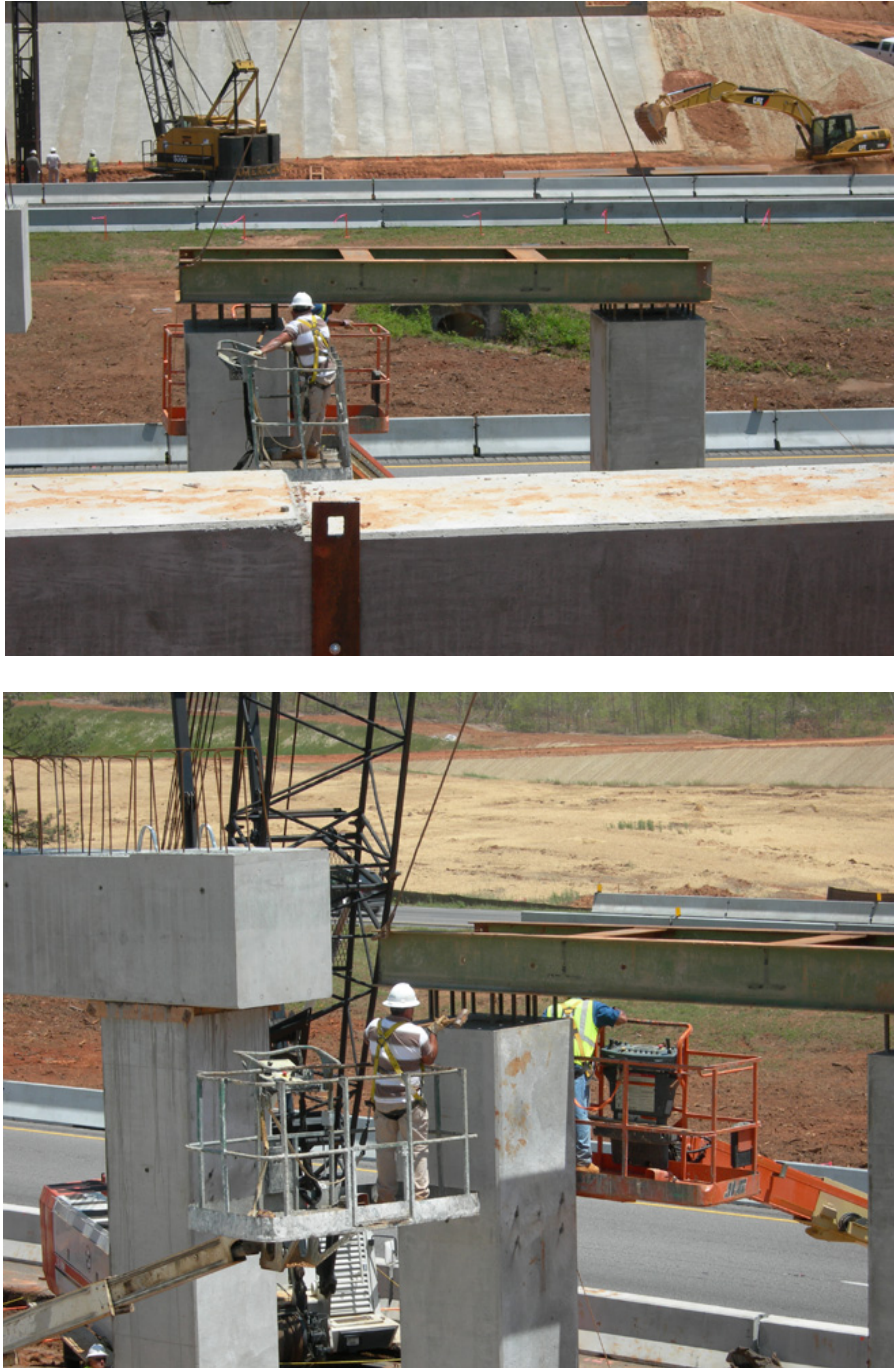
Figure 8. Workers check alignment of prefabricated columns with template.
