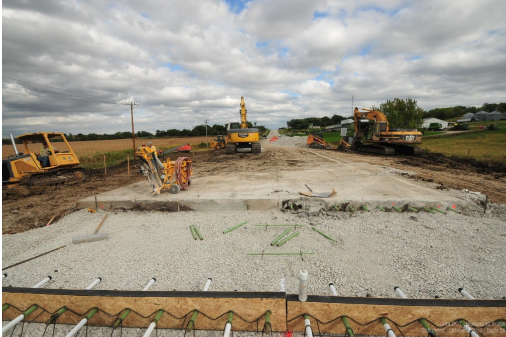
Figure 37. Photo. Approach connection (courtesy: Iowa DOT).
