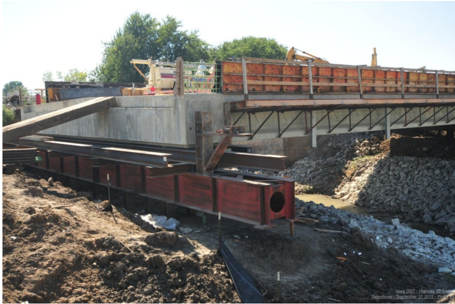
Figure 13. Photo. Completed superstructure (courtesy: Iowa DOT).
