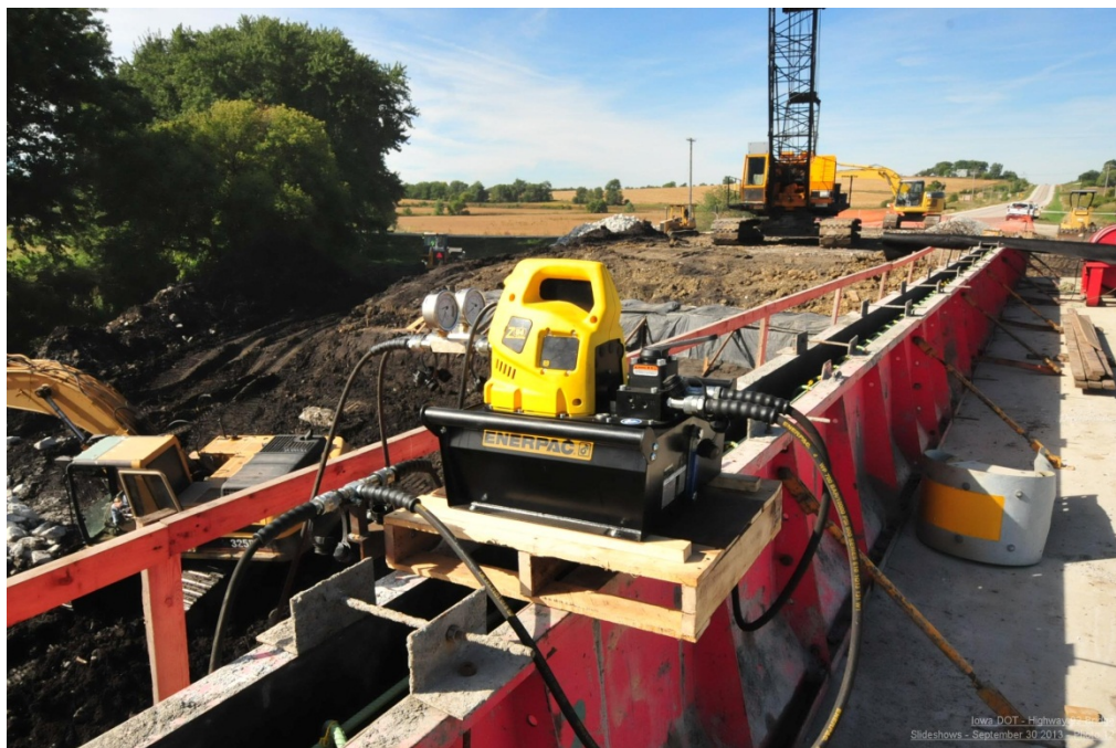
Figure 22. Photo. Slide jack control (courtesy: Iowa DOT).
