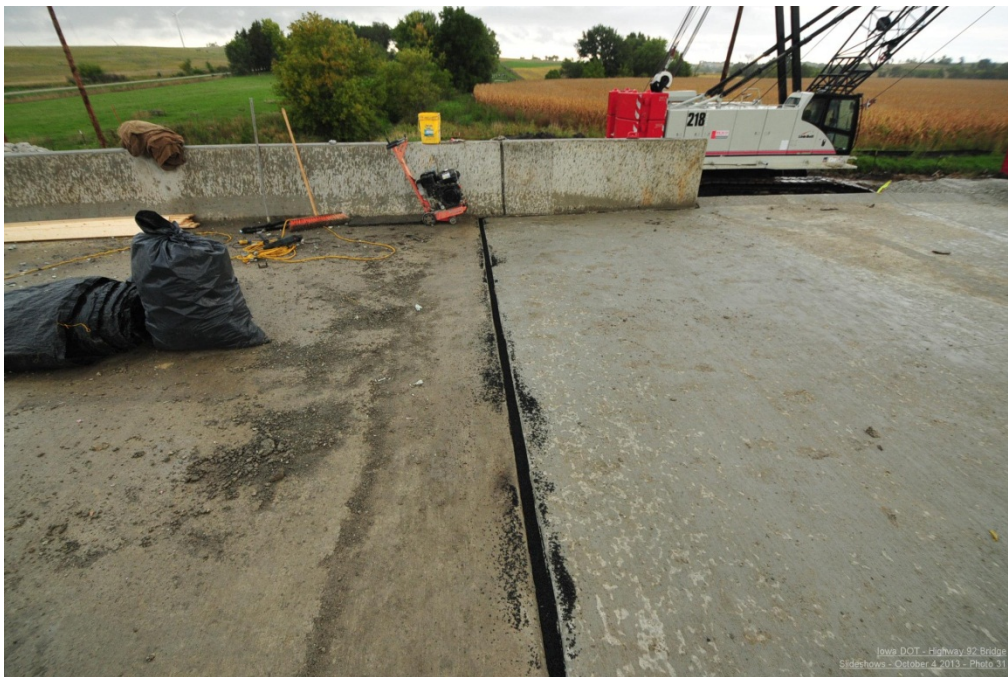
Figure 38. Photo. Expansion joint (courtesy: Iowa DOT).
