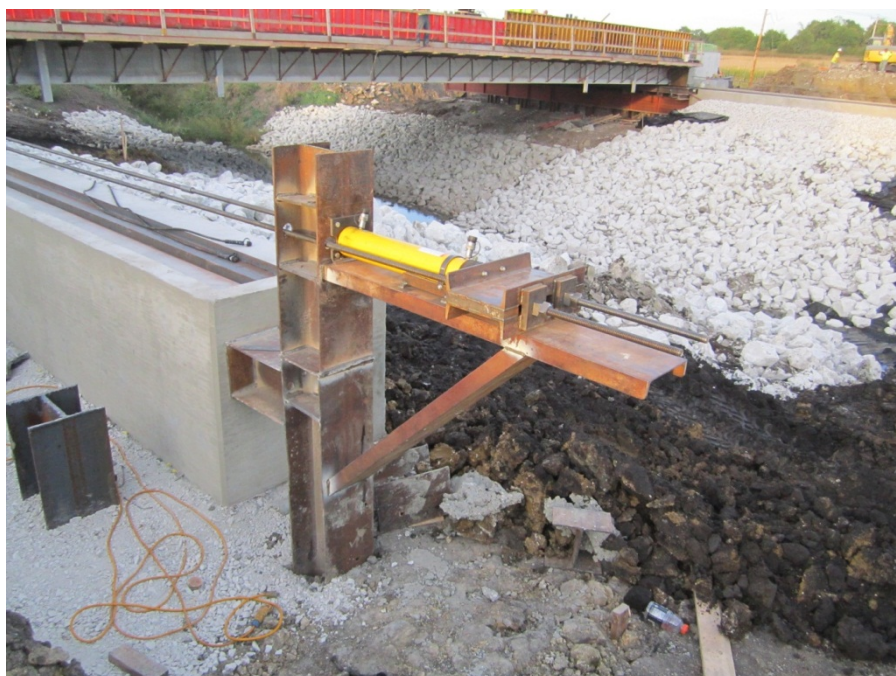
Figure 23. Photo. Jacking frame (courtesy: Iowa DOT).
