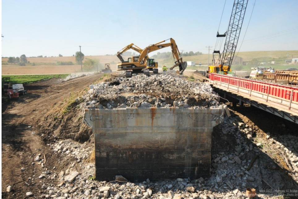
Figure 15. Photo. Bridge being demolished (courtesy: Iowa DOT).
