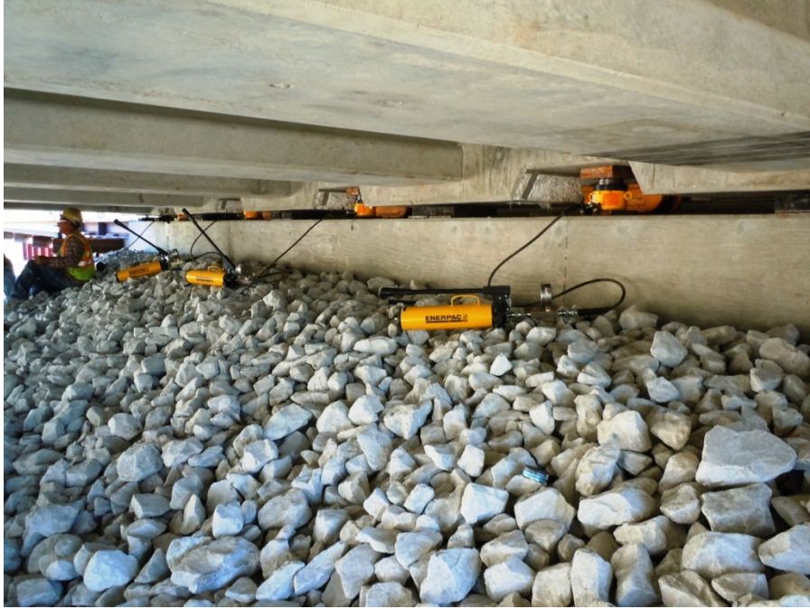
Figure 29. Photo. Bridge jacking (courtesy: Iowa DOT).
