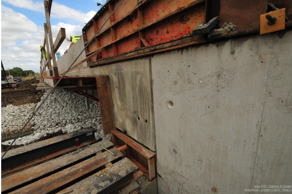
Figure 33. Photo. Bridge diaphragm and wing.
