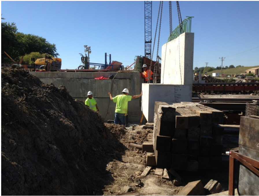
Figure 31. Photo. Precast wingwalls (courtesy: Iowa DOT).
