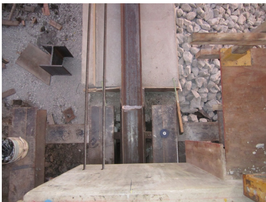
Figure 24. Photo. Slide transition (courtesy: Iowa DOT).
