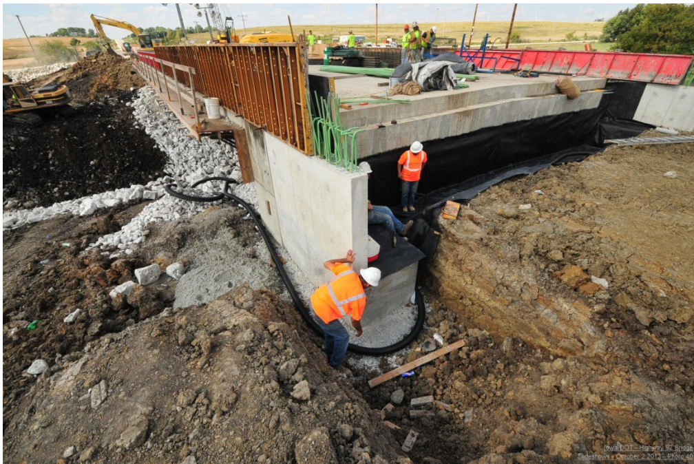
Figure 34. Photo. Subdrain (courtesy: Iowa DOT).
