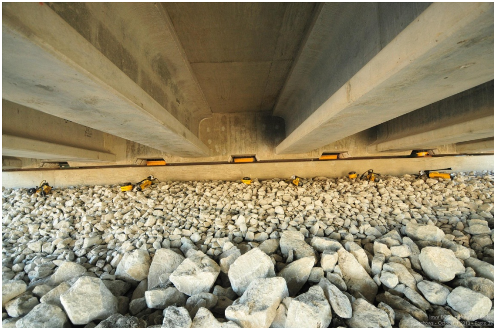
Figure 28. Photo. Roller removal (courtesy: Iowa DOT).
