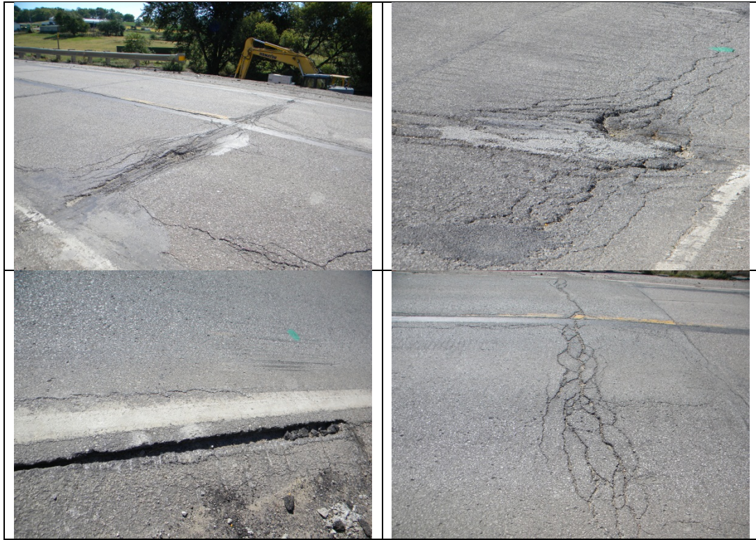
Figure 2. Existing Bridge Deck and Approach Roadway Conditions
