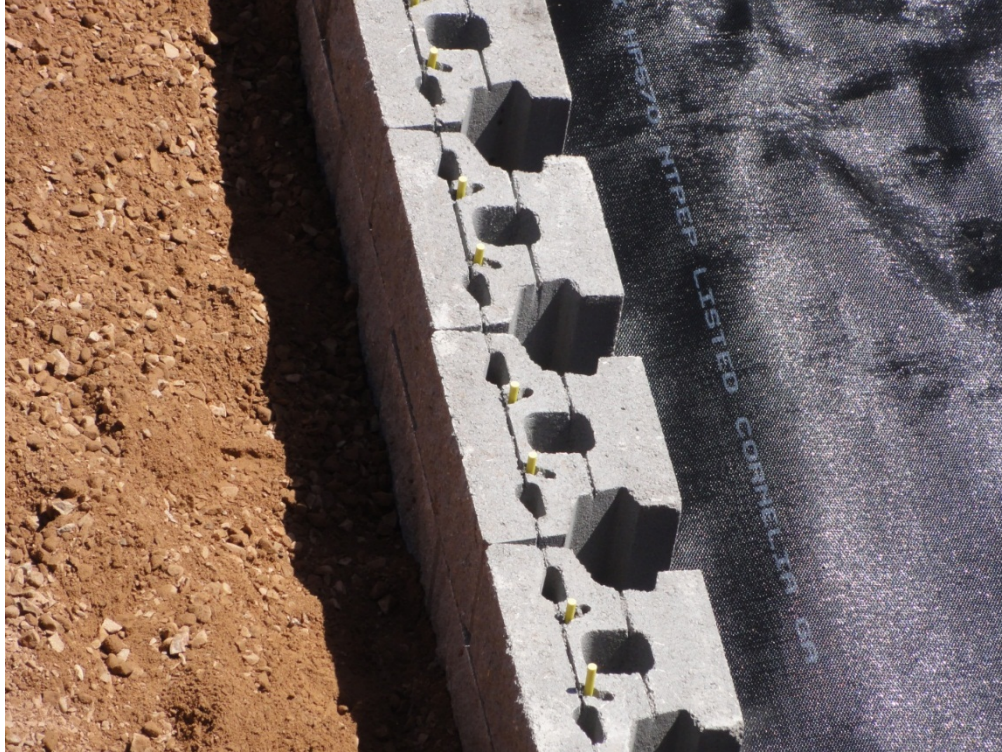
Figure 12. Photo. Segmental block units with fiberglass pins.
