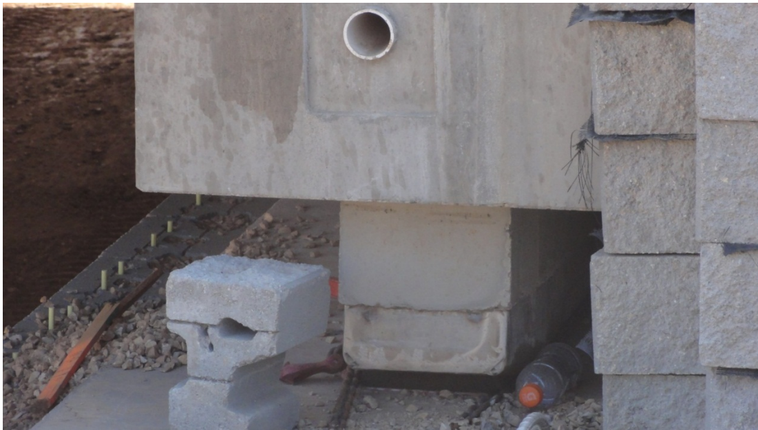
Figure 42. Photo. Slide shoe (side view).
