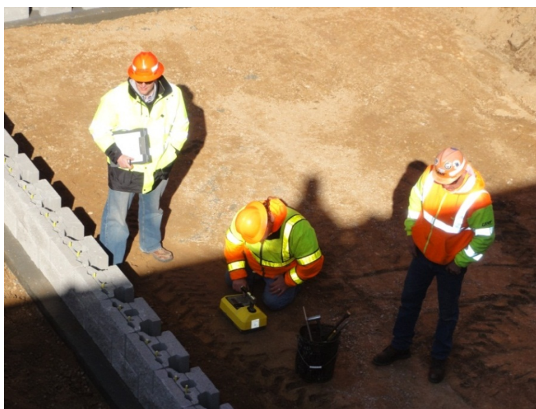
Figure 29. Photo. Density measurements being taken.
