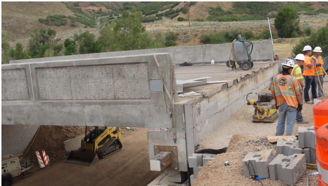
Figure 52. Photo. Bridge slide completed.
