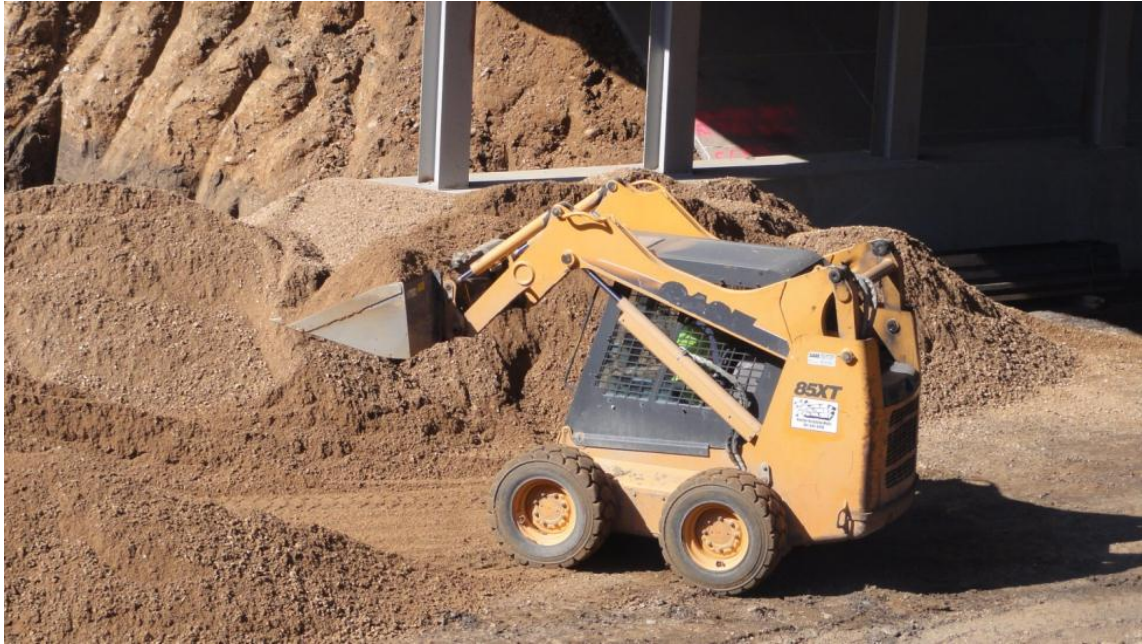
Figure 23. Photo. Soil being distributed across the site.
