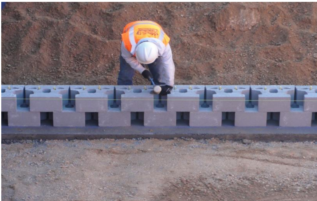
Figure 27. Photo. Aligning the second course or SMU blocks.
