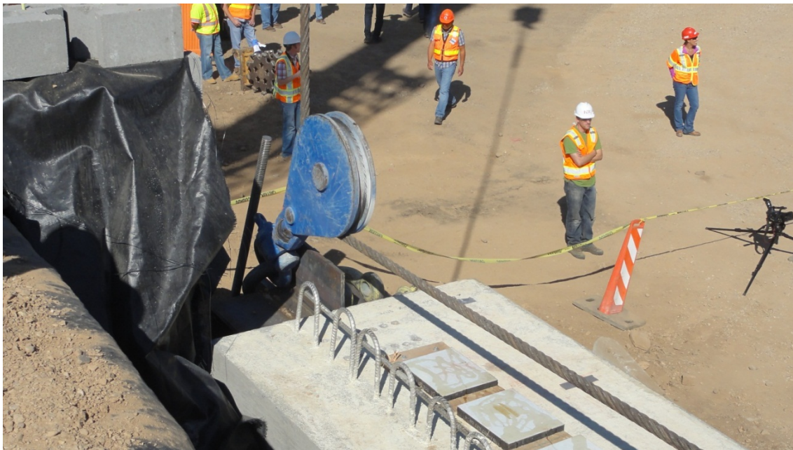
Figure 46. Photo. Snatch block connecting to the cable.
