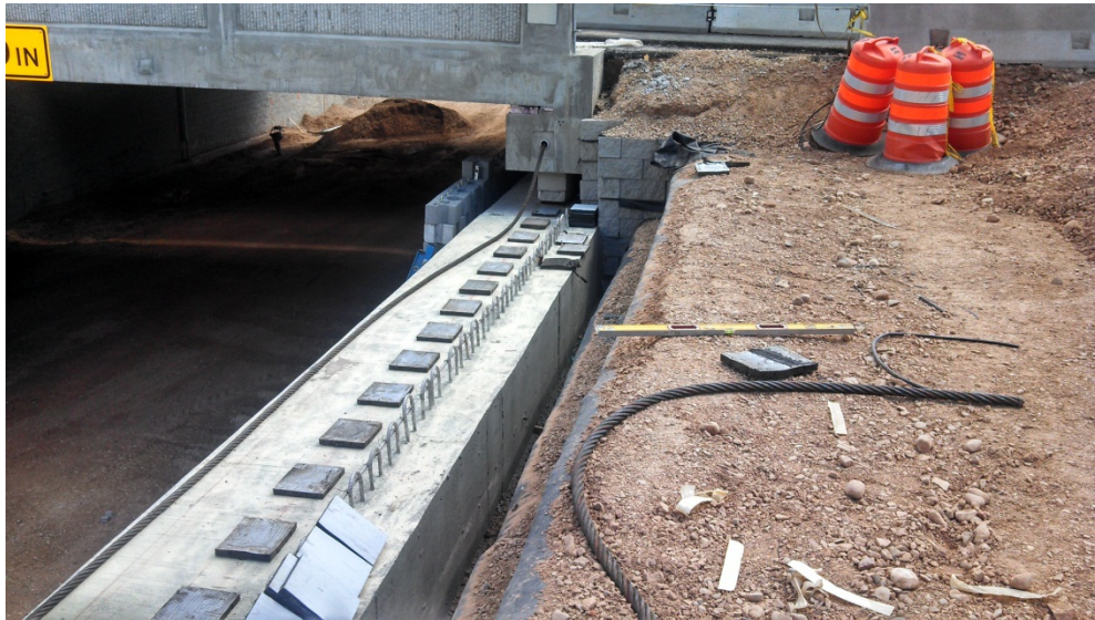
Figure 43. Photo. Neoprene pads for slide (courtesy: UDOT).
