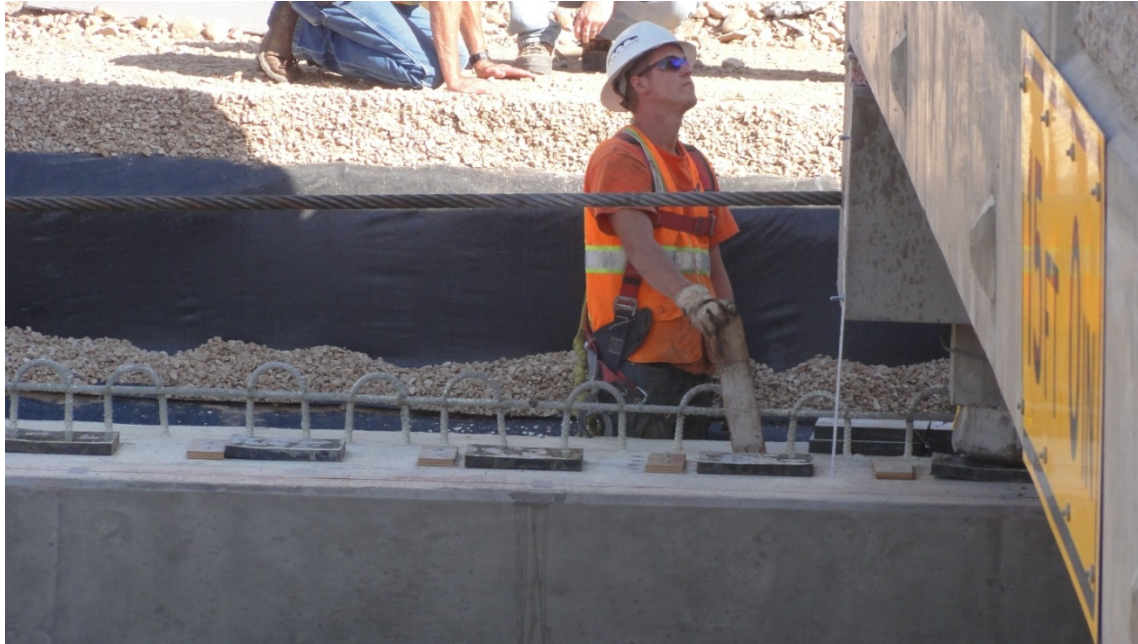
Figure 51. Photo. Bridge being slid across.
