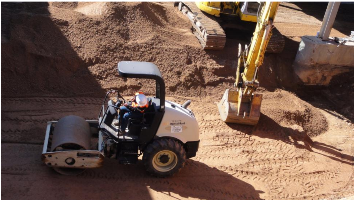
Figure 24. Photo. Roller operations.
