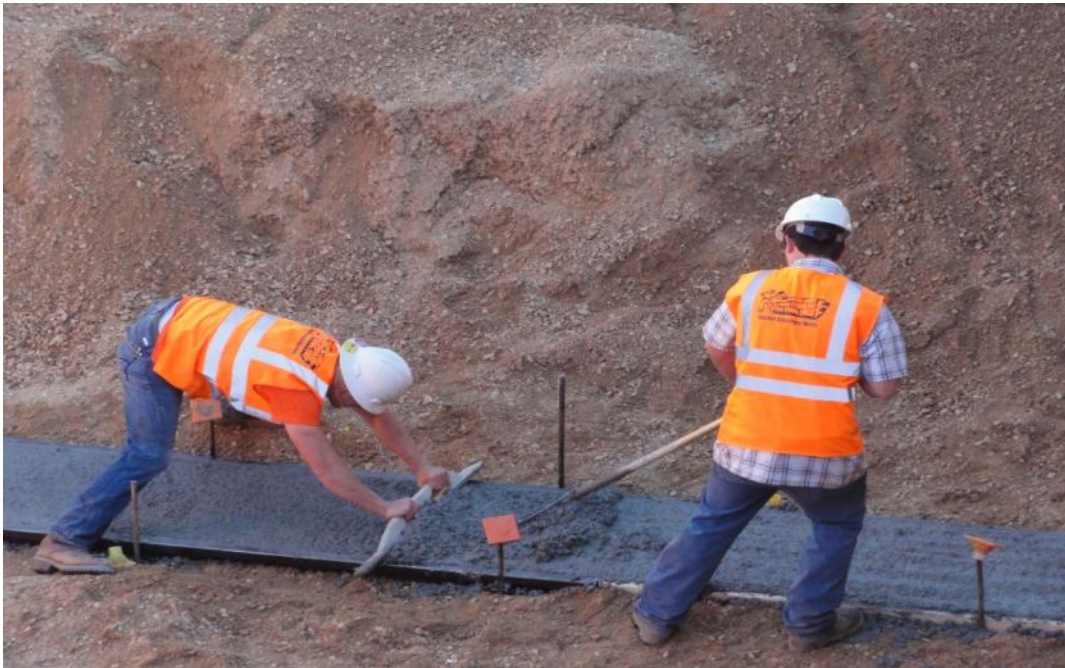
Figure 26. Photo. Preparation of leveling pad.
