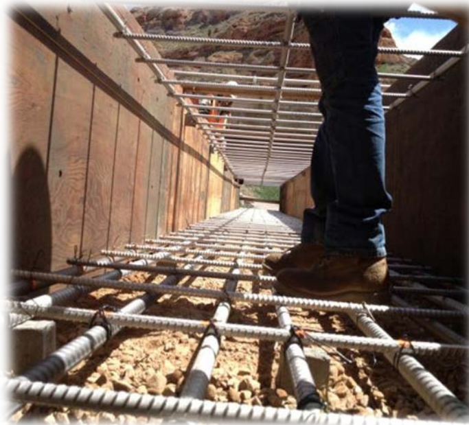
Figure 34. Photo. Bearing sill/footing (courtesy: UDOT).
