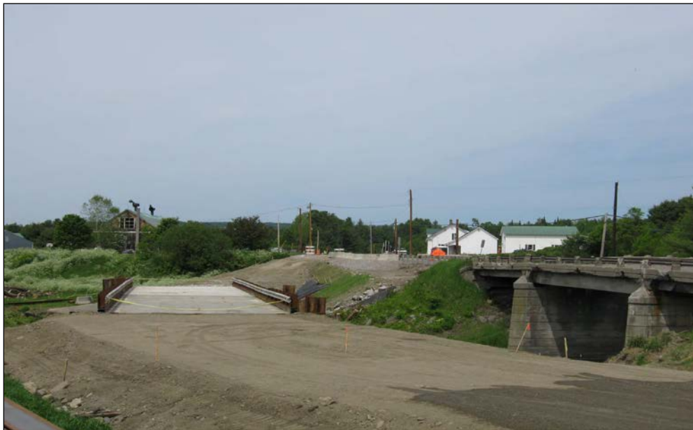
Figure 17. Construction of two-way temporary bypass bridge.
