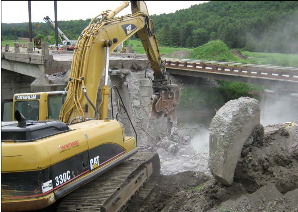
Figure 18. Demolition of the existing bridge.
