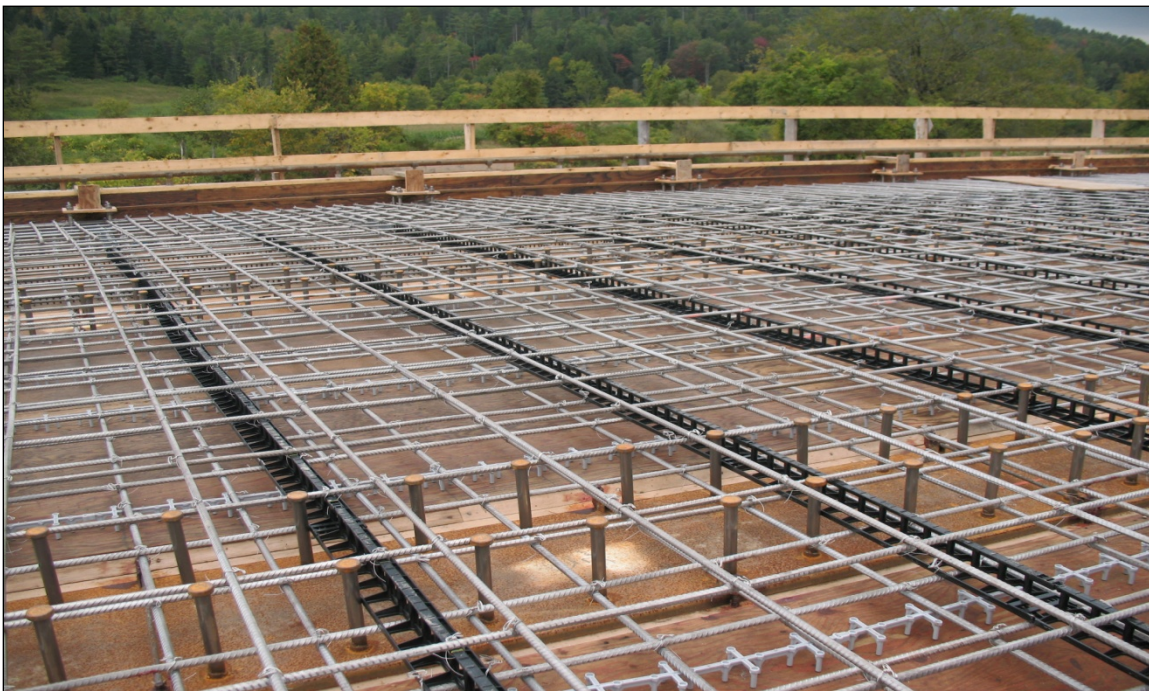
Figure 25. Close-up of deck reinforcement.
