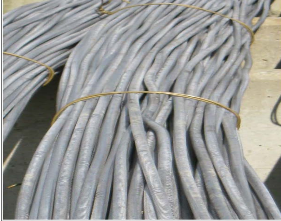
Figure 21. Close-up of stainless steel rebar condition.
