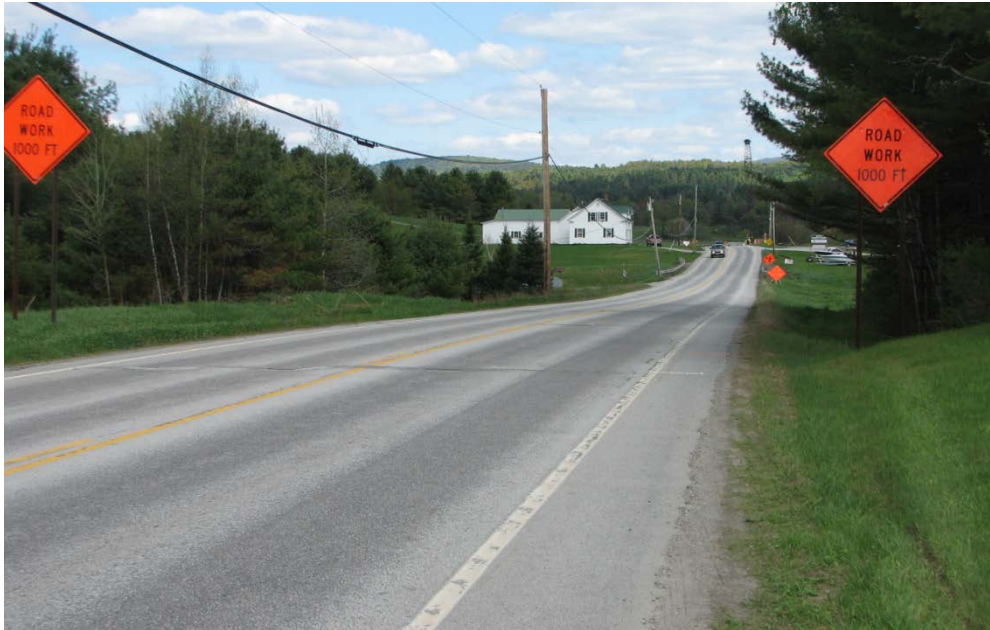
Figure 30. First work zone warning.
