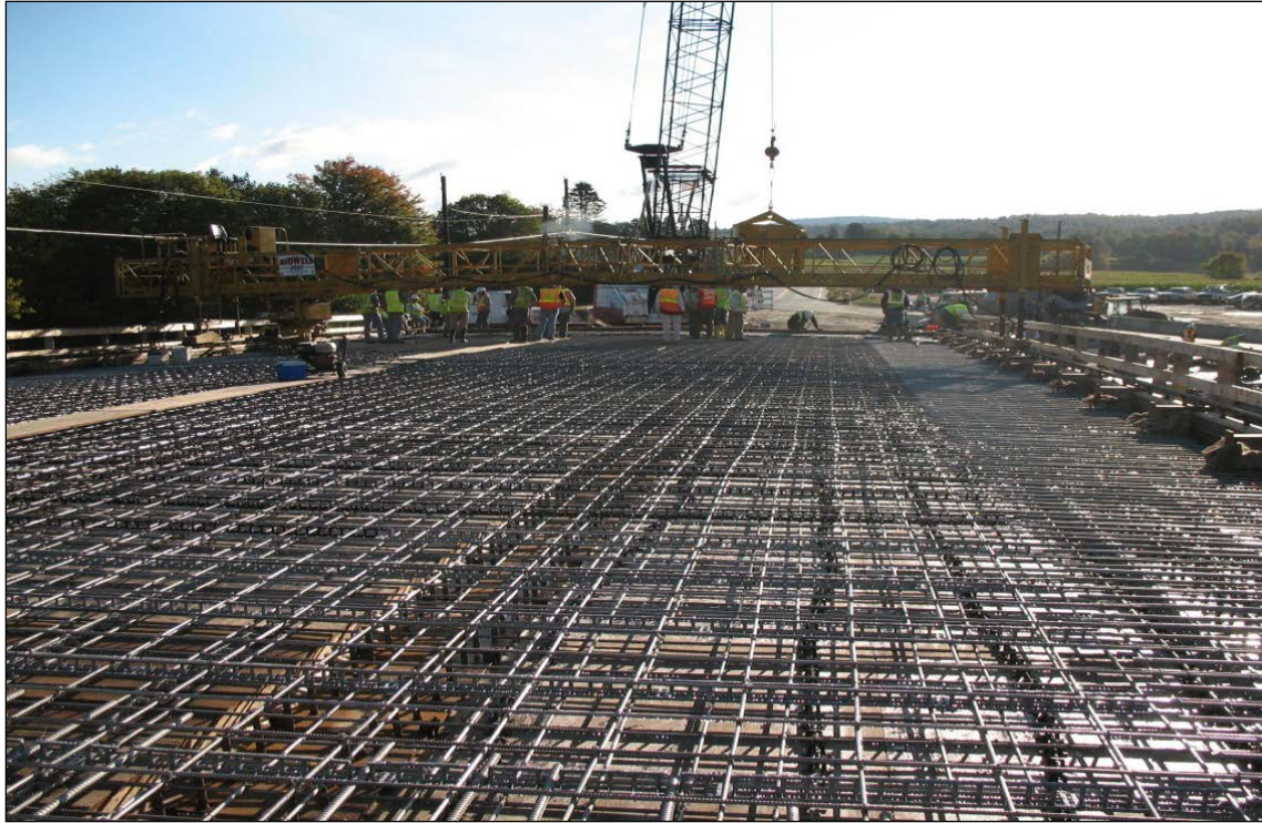
Figure 24. View of deck reinforcement.
