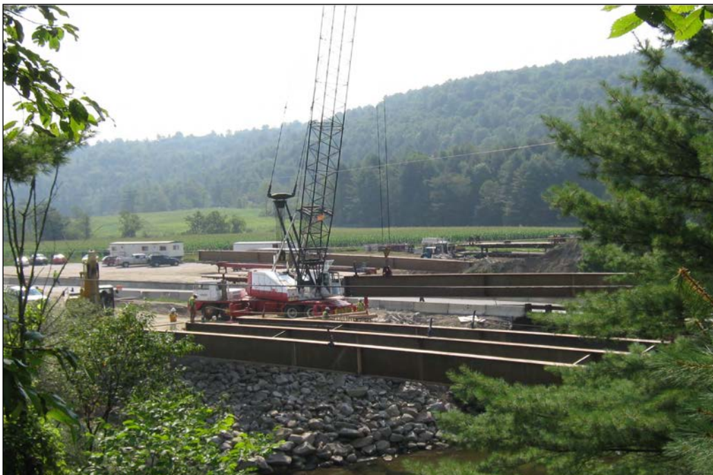
Figure 19. Placement of weathering steel girders.
