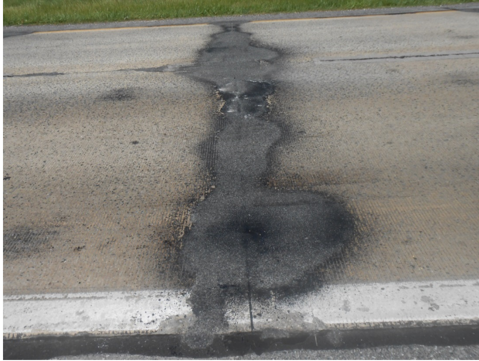
Figure 7. Photo. Full-width spray patching on Delaware LTPP test section 10_0208.
