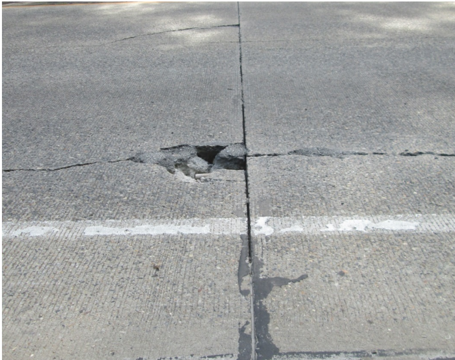
Figure 6. Photo. Cracking and spalling on Arkansas LTPP test section 05_0217.
